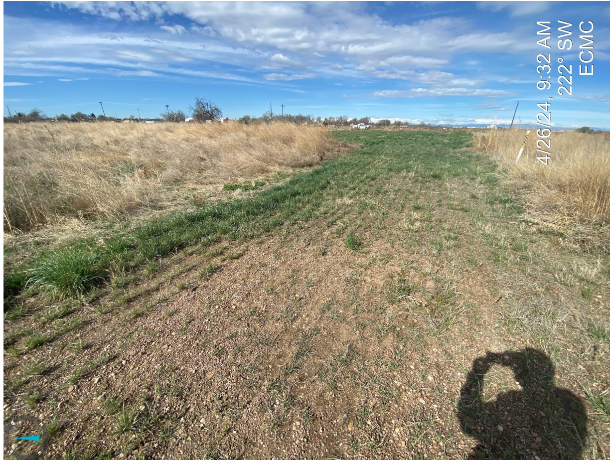
Photo 1. An area along the access road has evidence of road base material and non-uniform vegetation cover; additional reclamation activities are required.
