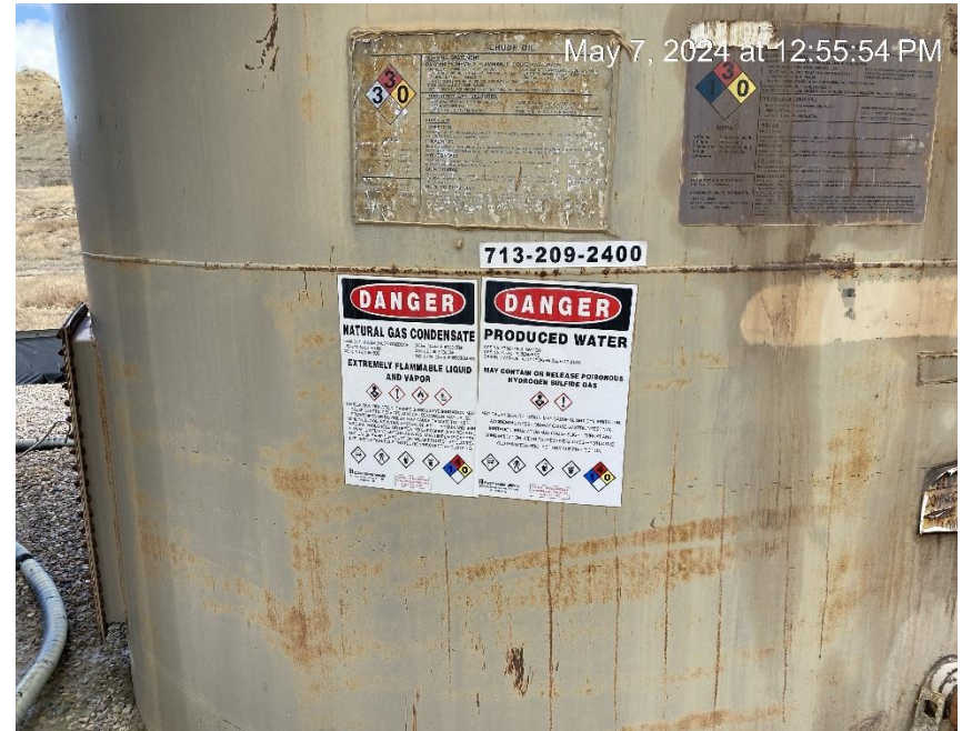
Tank label missing required information
