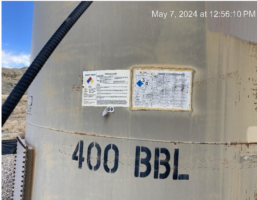
Tank label missing required information
