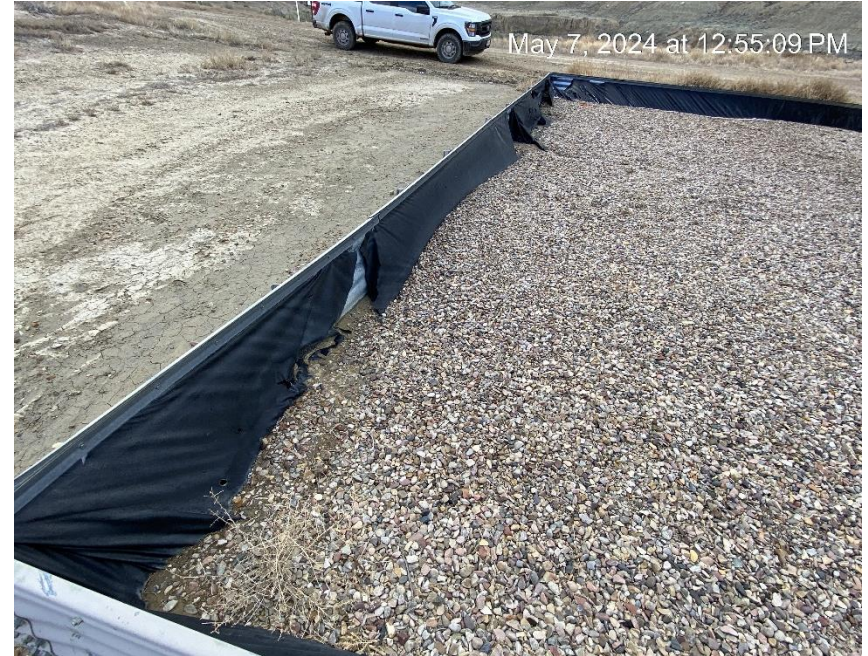
Liner no longer impervious to fluids
