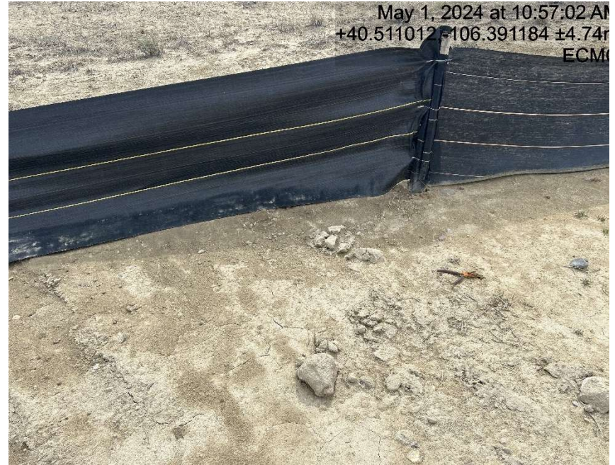
Silt fence failing
