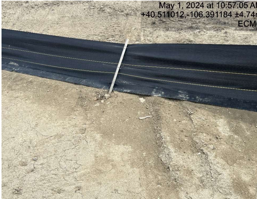
Silt fence failing
