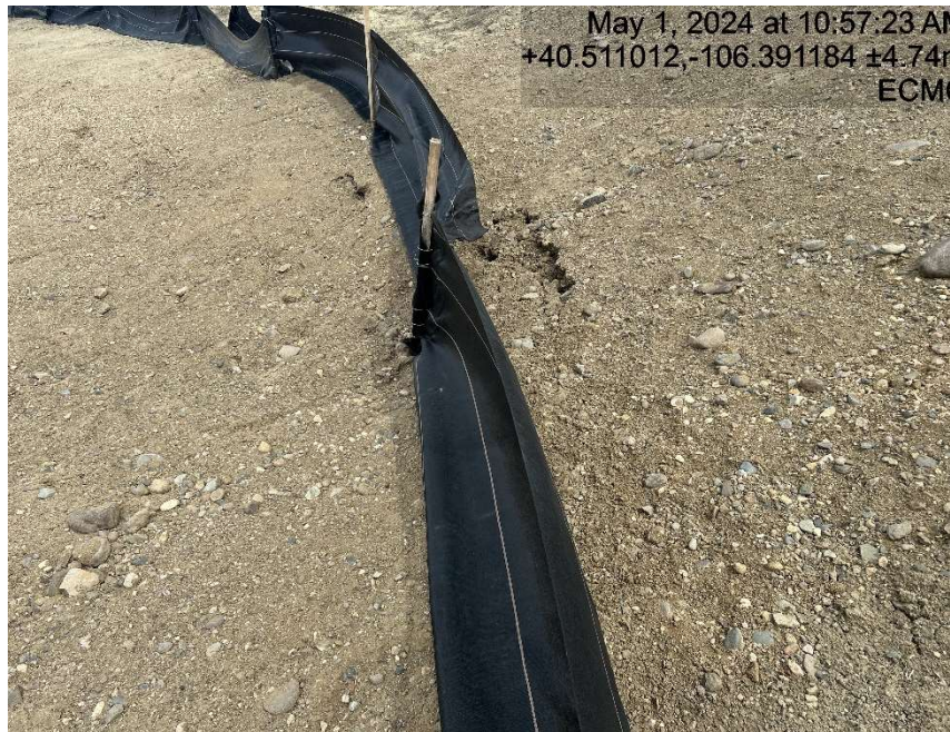
Silt fence failing
