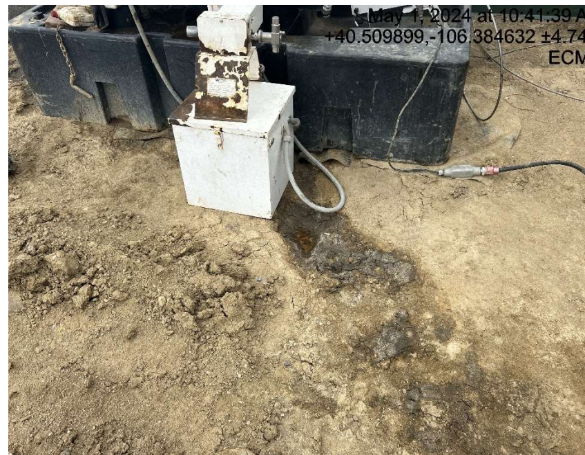
Staining coming from under chemical tank containment
