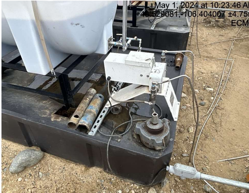
Debris and chemical containment full of fluid
