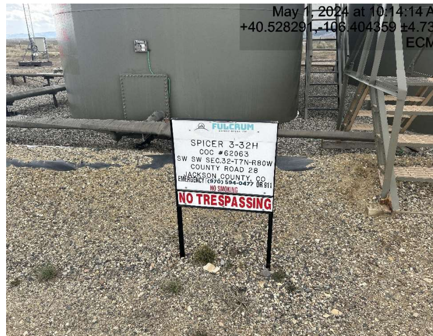
Battery sign lacking API's
