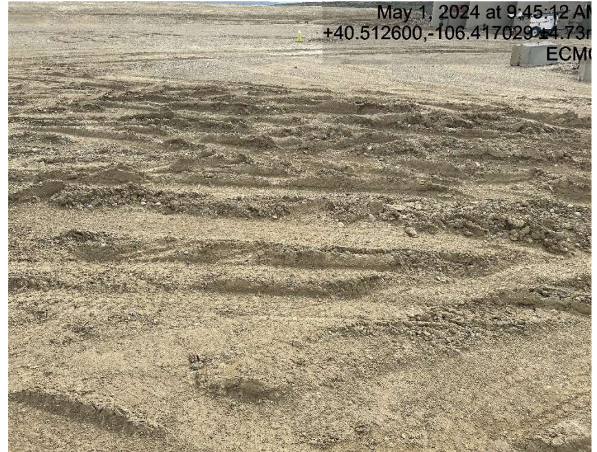
Lack of stabilization/compaction
