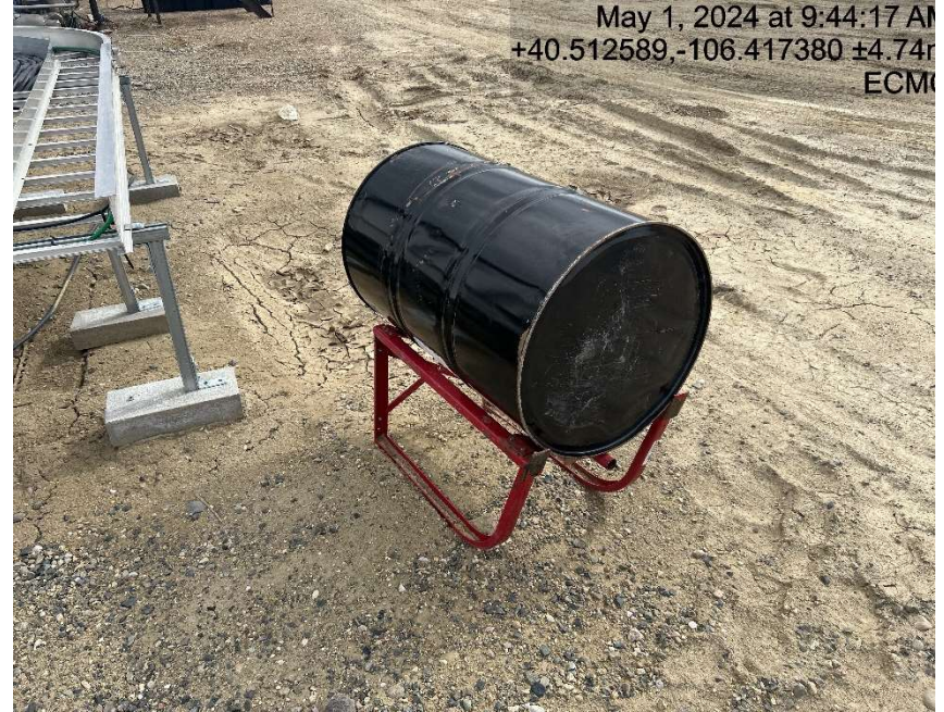
Unknown tank and not in secondary containment
