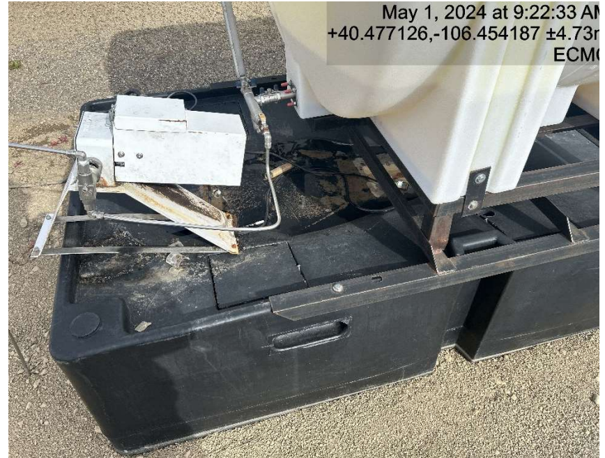
Chemical containment is full of fluid
