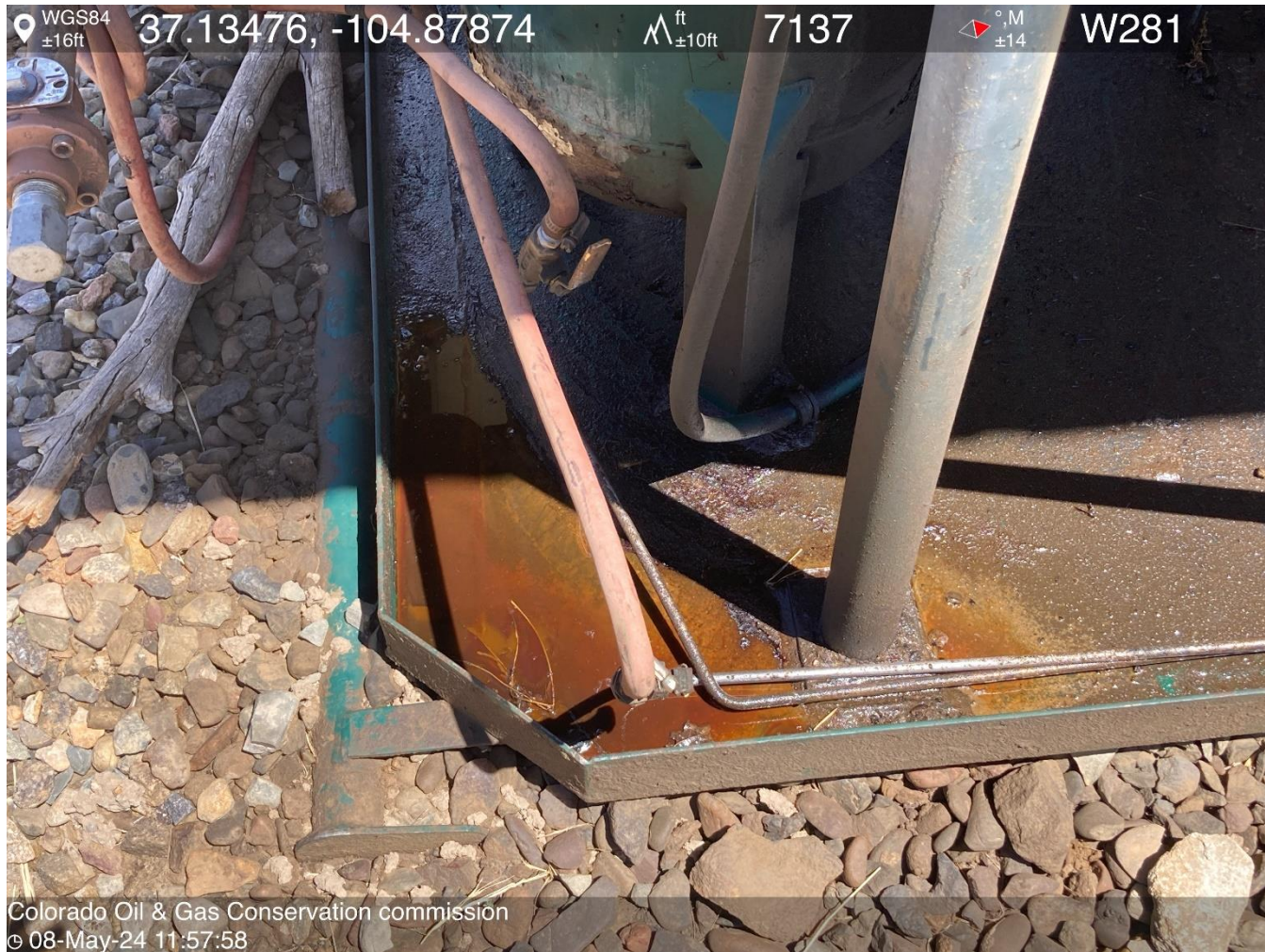
PHOTO 8: OILY WASTE IN ENGINE SKID. COMPLY WITH RULE 1002.f.(2)B, Comply with general provisions of the oil and gas act for wildlife protection AND SB-181. CA DATE 5-9-2024.
