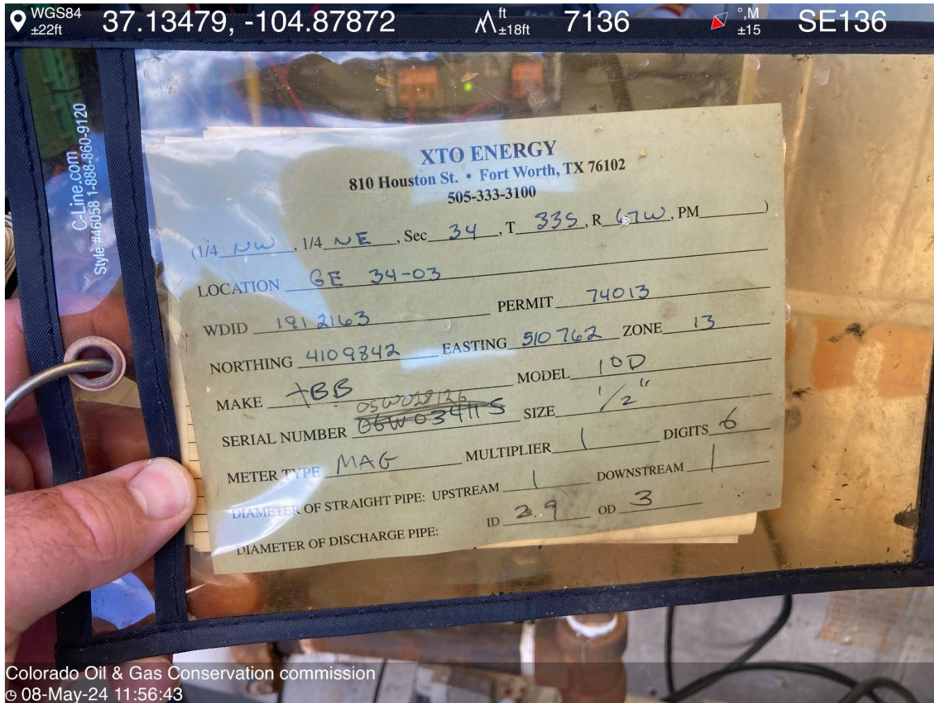
PHOTO 7: NO CURRENT CALIBRATION LOG POSTED AT METER. PROVIDE AREA FIELD INSPECTOR (@ tombeardslee@state.co.us) A COPY OF THE GAS METER CALIBRATION RECORD OR KEEP A COPY OF LAST CALIBRATION RECORD ON LOCATION. CA DATE 6-8-2024.
