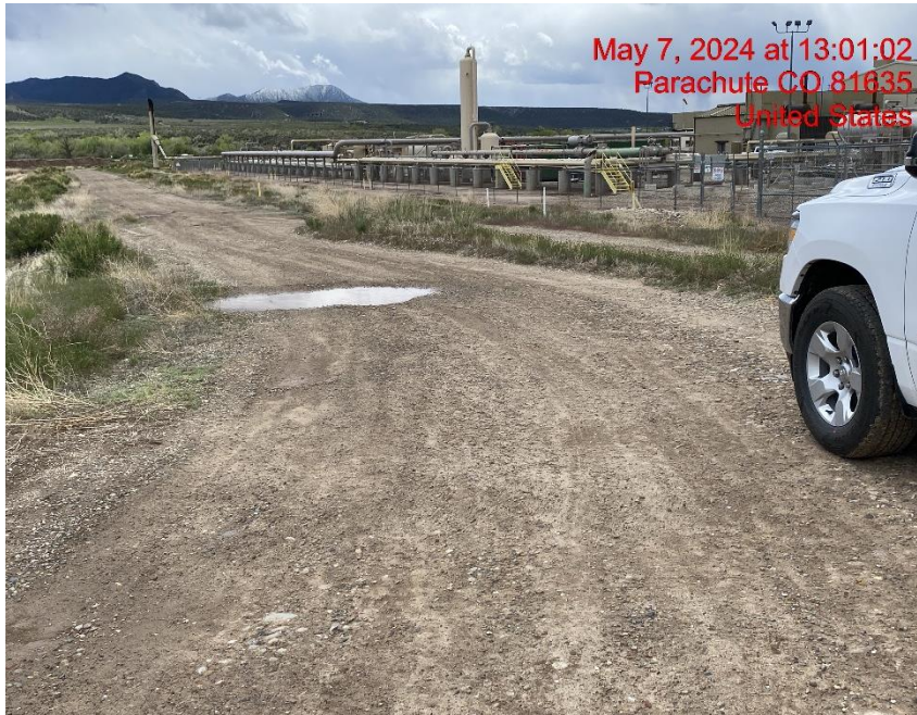
Insufficient Vehicle Tracking BMPs at Location Entrance/Exit – Photo #00972
