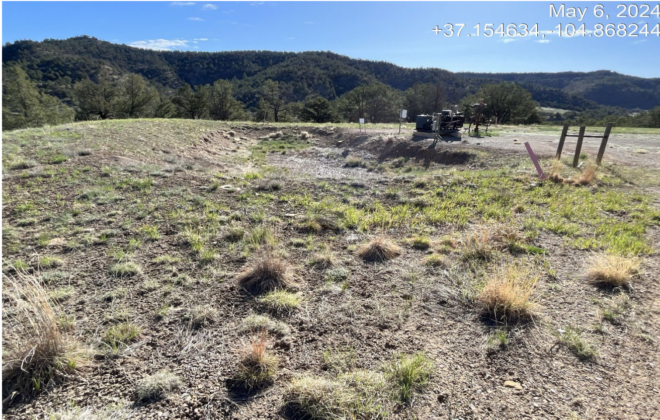
Photo 2. Facing northeast toward the production pit.
