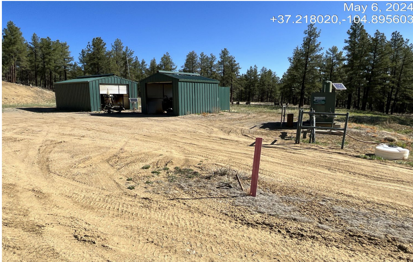
Photo 2. Facing northeast at the wellsite.
