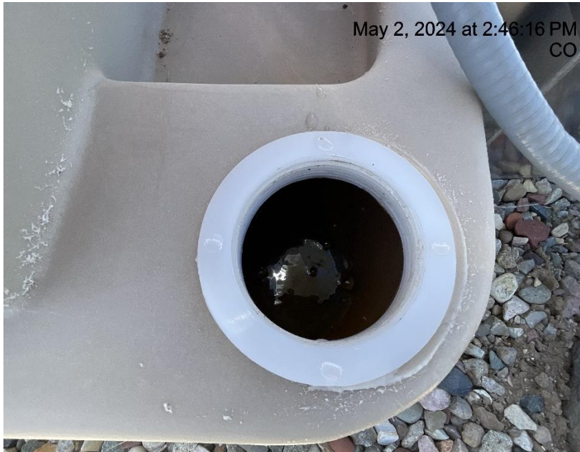
Photo # 5659 From inspection 708903684 conducted on 05/02/2024 Failure to maintain chemical BMP/chemical containment approximately 3/4 full of fluid/BMP insufficient to contain possible spill.
