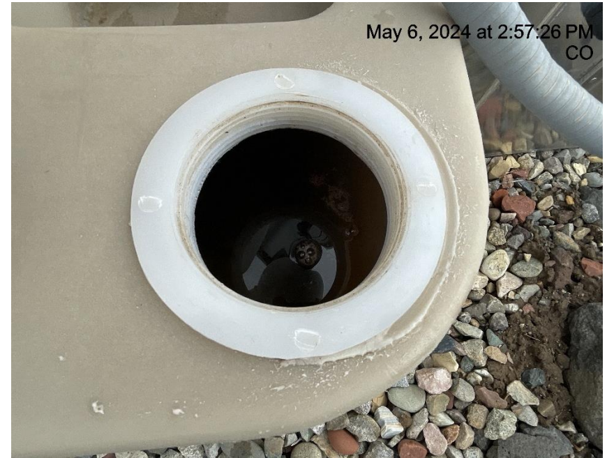
Photo # 6015 Failure to maintain chemical BMP/chemical containment approximately 3/4 to 7/8 full of fluid/BMP insufficient to contain possible spill.
