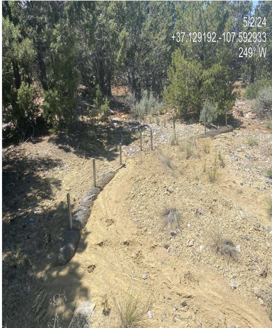
Photo 3. Failing storm water BMPs observed in the western interim reclamation area, maintenance is required.
