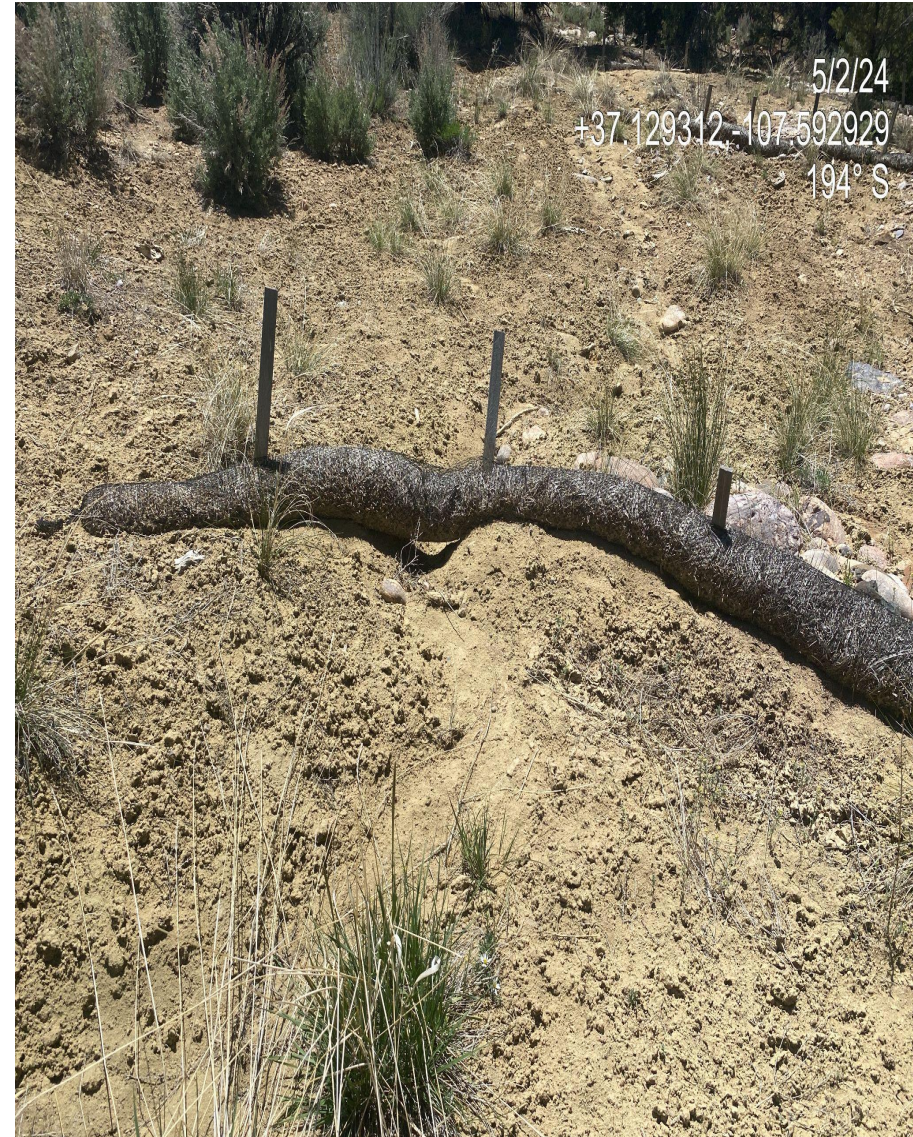
Photo 3. Failing storm water BMPs observed in the western interim reclamation area, maintenance is required.
