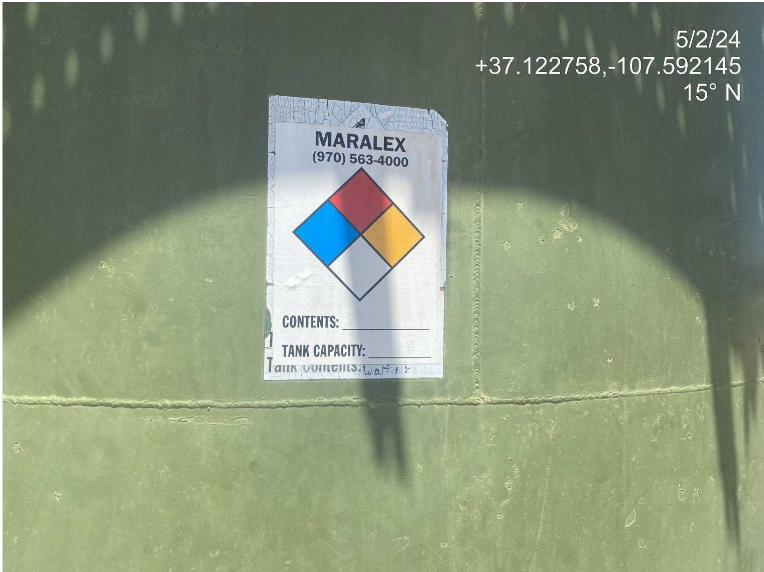
Photo 5. Capacity not listed at tank battery produced water tanks.
