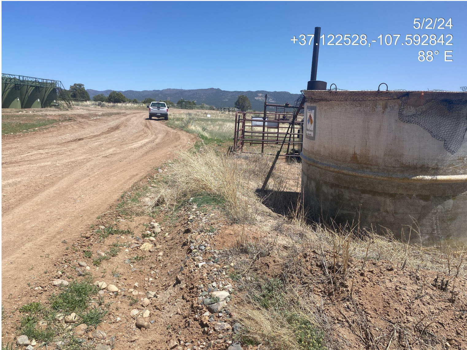
Photo 3. Weedy debris at produced water tank berm have not been removed. Maintenance on secondary containment is required.
