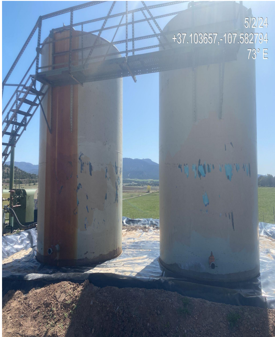
Photo 3. Produced water tanks on location are in use but are not marked.
