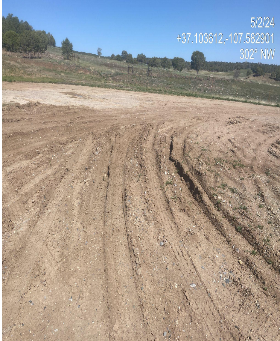
Photo 5. View of rutting observed on the active pad. Additional stabilization is needed to minimize site degradation.
