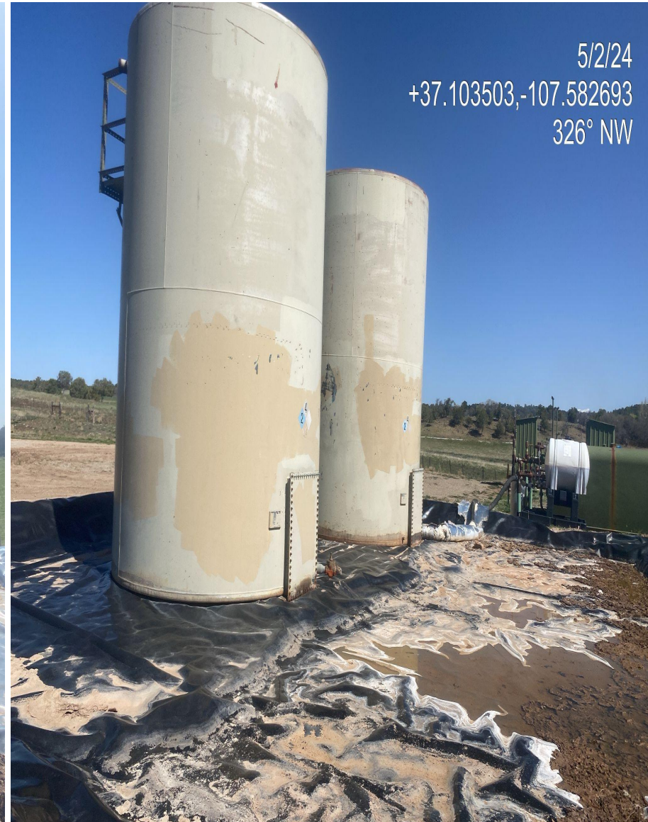
Photo 3. Produced water tanks on location are in use but are not marked.
