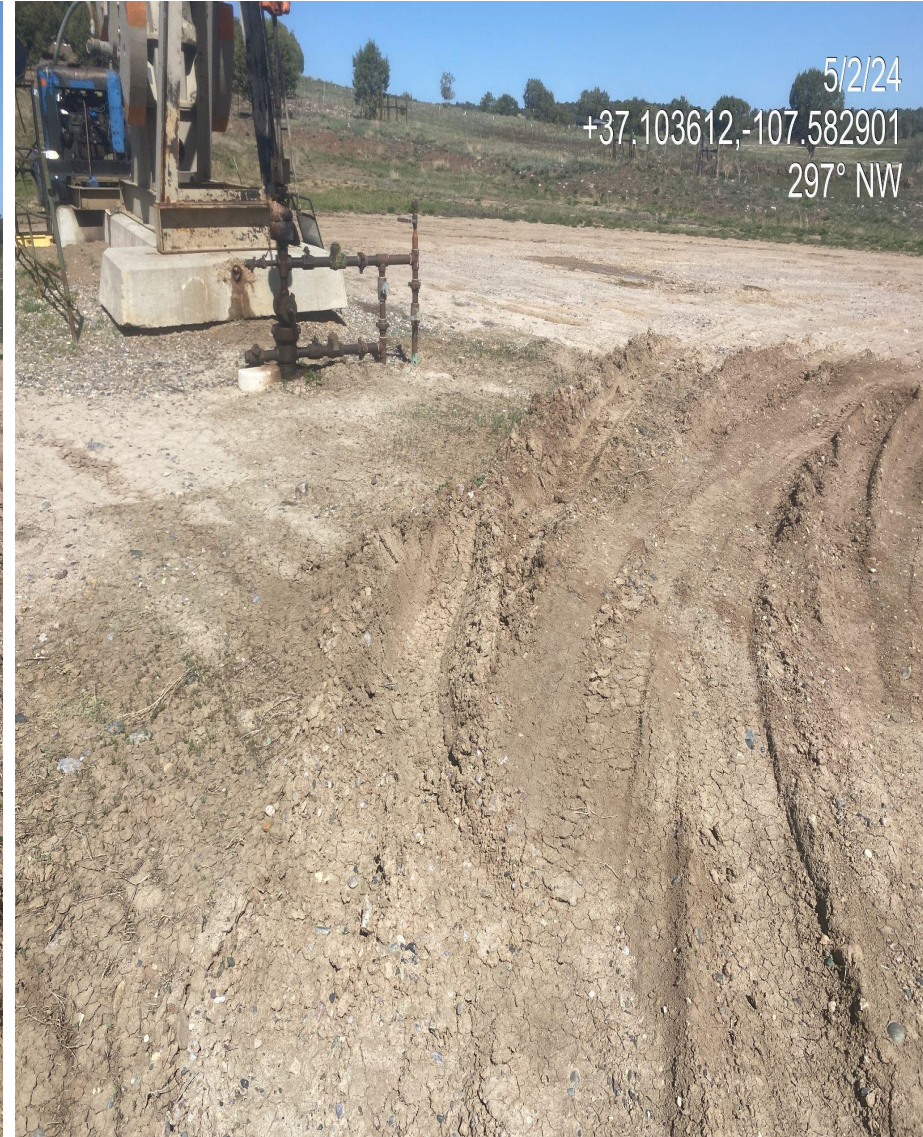
Photo 5. View of rutting observed on the active pad. Additional stabilization is needed to minimize site degradation.
