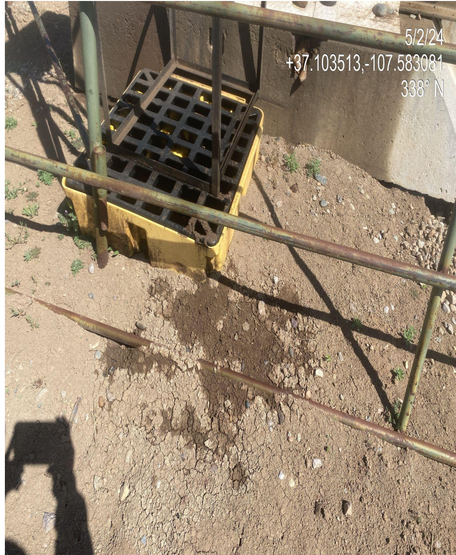
Photo 7. View of impacted surface material at both lube oil tanks secondary containments at both pump jacks.
