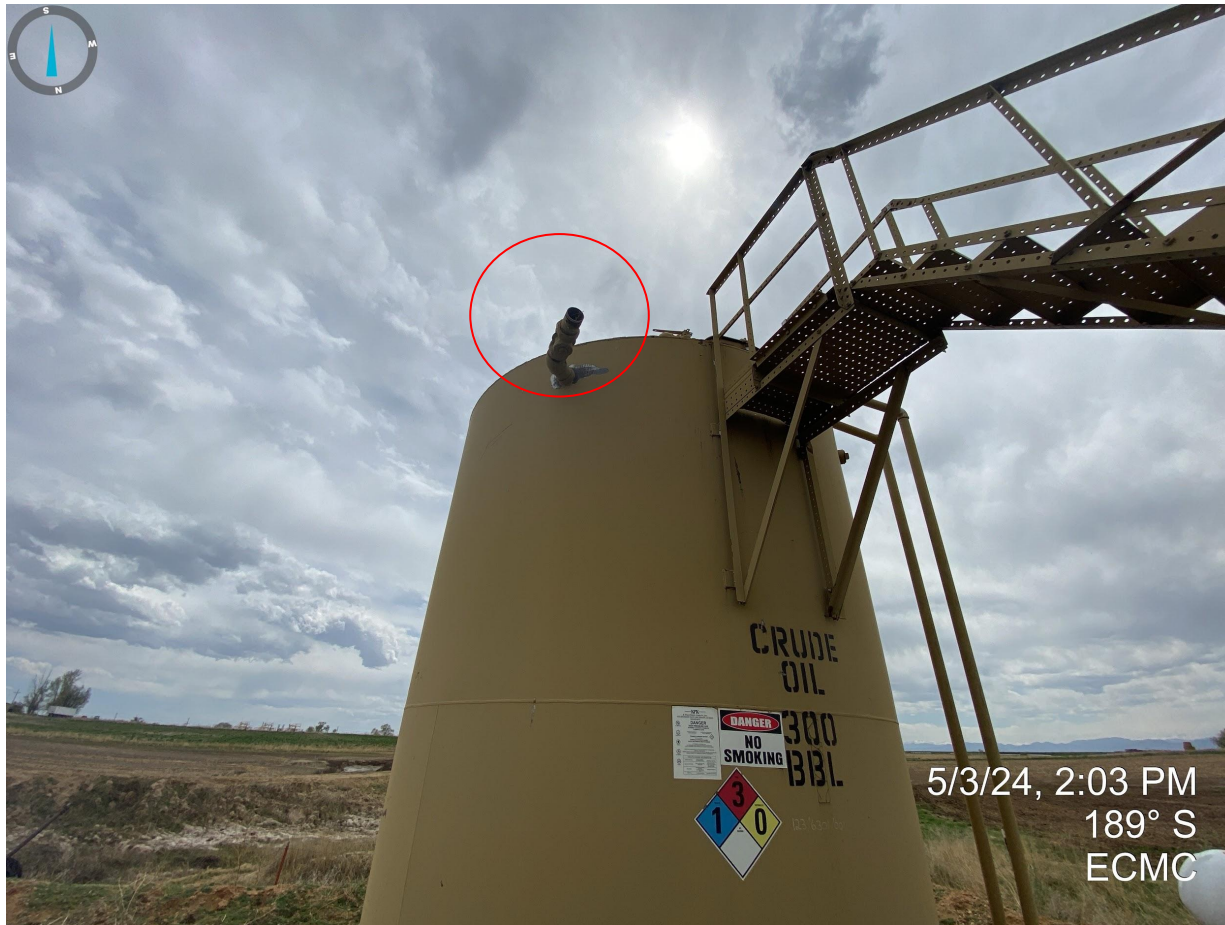
Photo 18. Tank battery does not have adequate wildlife exclusion devices installed at openings.
