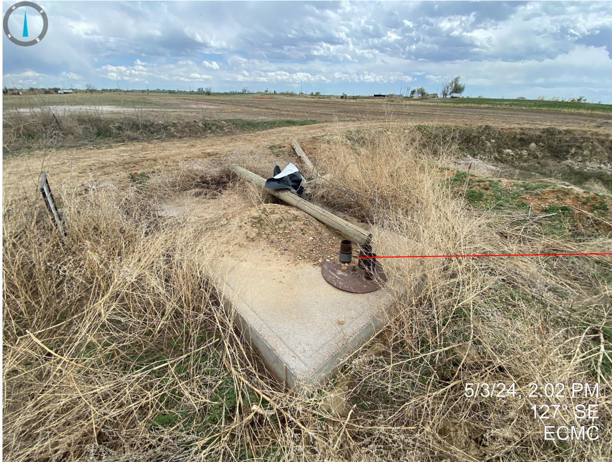
Photo 14 & 15. Buried produced water vault does not have adequate wildlife exclusion devices installed at openings.
