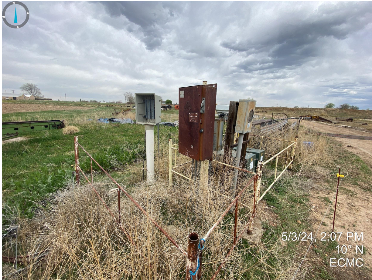
Photo 21. Weed debris observed throughout production equipment (electrical panels).
