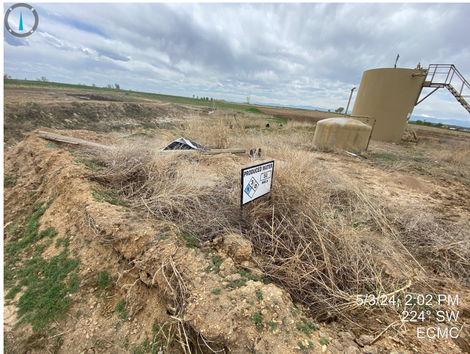
Photo 12 & 13. Secondary containment/berms around tank battery facility is not adequate as evidenced by unconsolidated materials and damage to berms (right photo, red arrow). Debris, trash and undesirable vegetation (kochia) also observed throughout.
