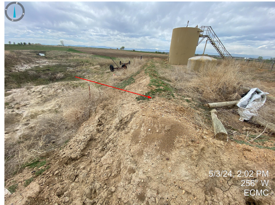
Photo 12 & 13. Secondary containment/berms around tank battery facility is not adequate as evidenced by unconsolidated materials and damage to berms (right photo, red arrow). Debris, trash and undesirable vegetation (kochia) also observed throughout.
