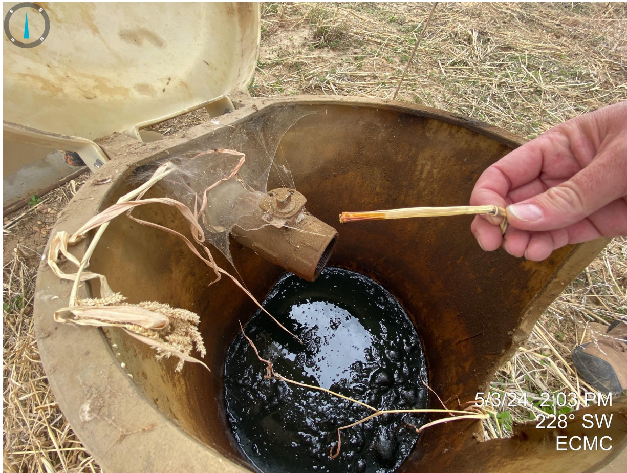
Photo 19. Free fluids observed within loadout line collection bucket need to be properly cleaned and disposed of.
