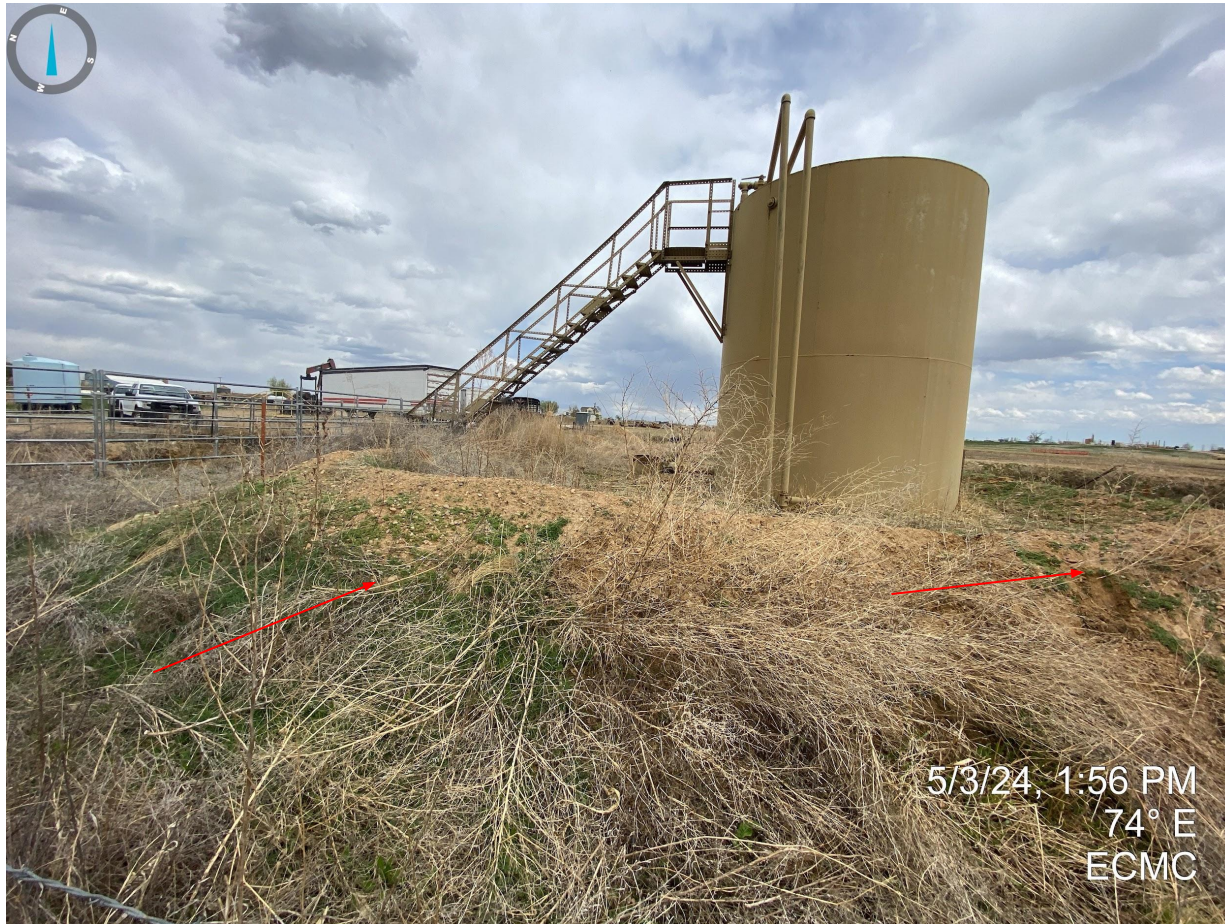
Photo 2. Undesirable vegetation (kochia) growing throughout the tank battery secondary containment.
