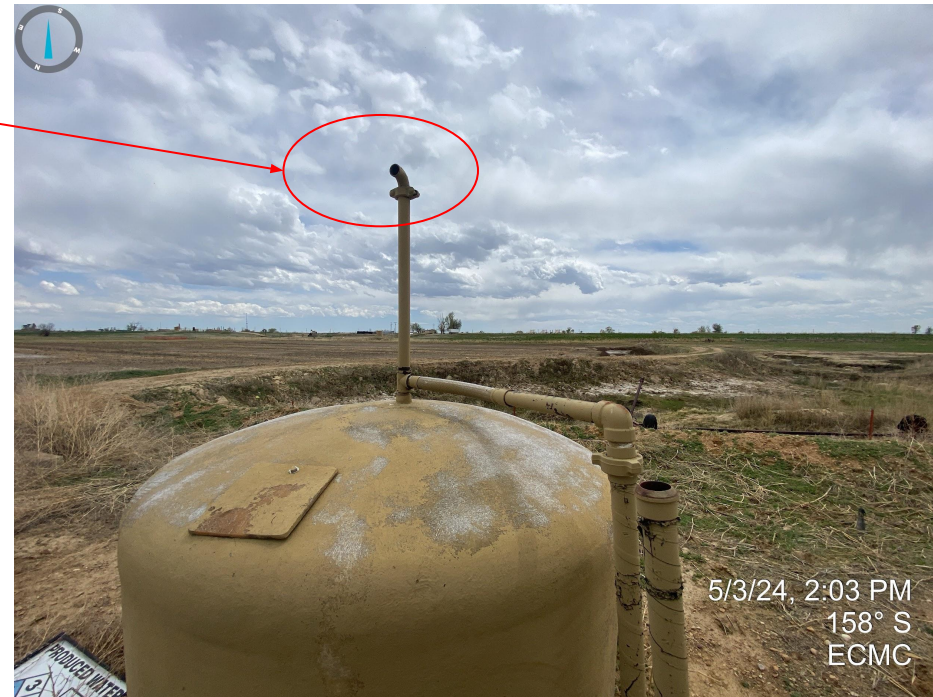
Photo 16 & 17. Fiberglass tank does not have adequate wildlife exclusion devices installed at openings.
