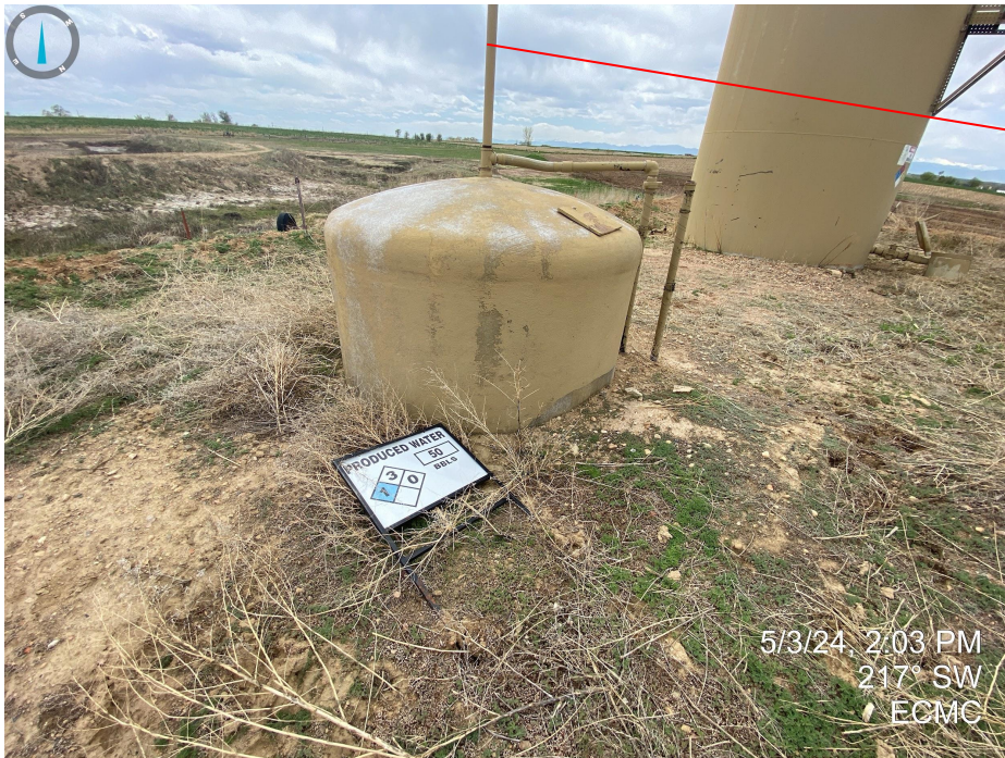
Photo 16 & 17. Fiberglass tank does not have adequate wildlife exclusion devices installed at openings.
