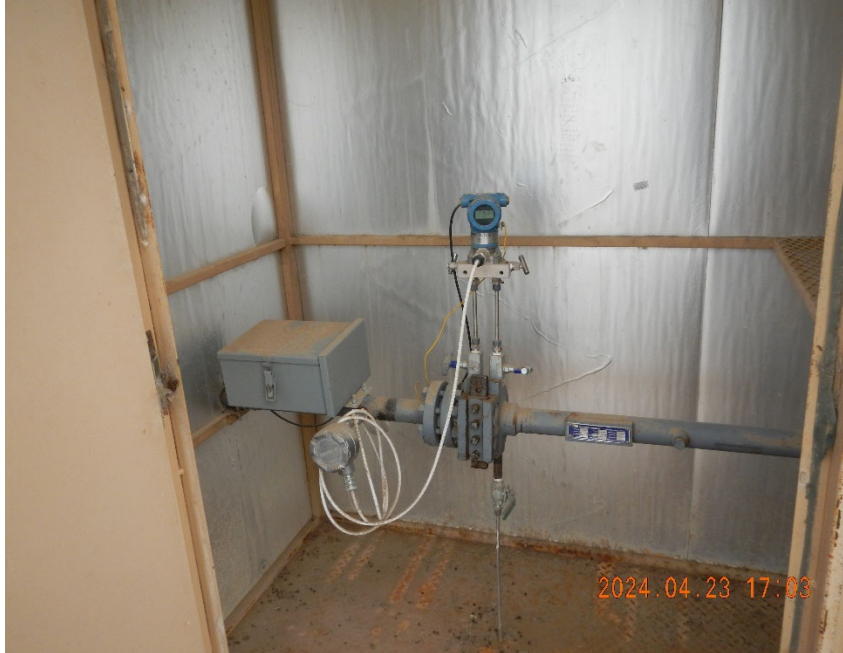
3. Digital gas meter inside meter shed.
