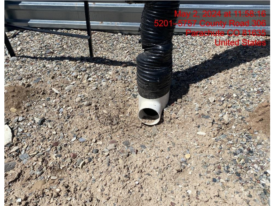
Open-Ended Heating Line – Photo #00932
