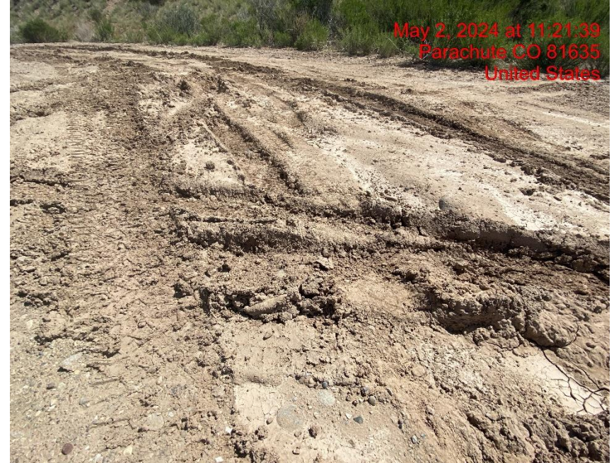
Lack of Stabilization – Photo #00915
