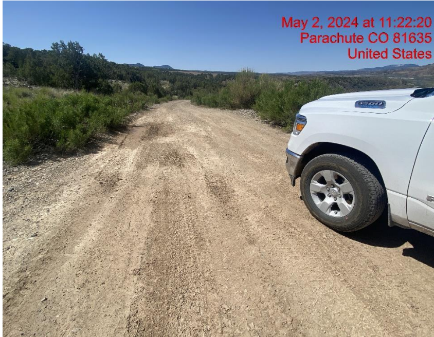
Insufficient Vehicle Tracking BMPs at Location Entrance/Exit – Photo #00916
