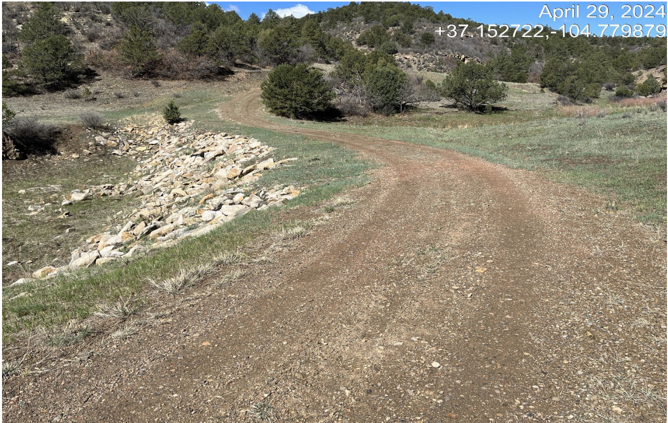
Photo 2. Facing west along the access road. The drainage crossing is stabilized with BMP's
