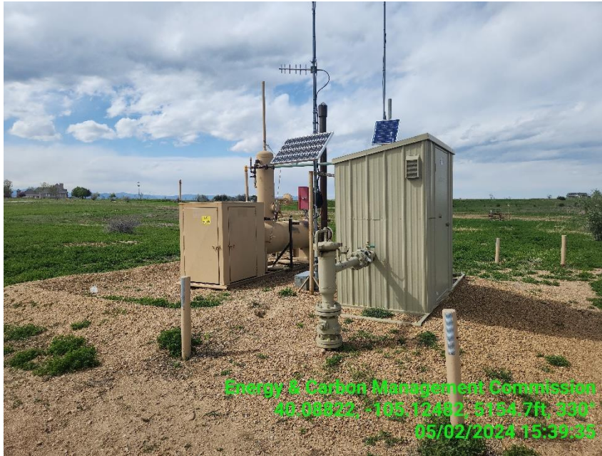
Photo 5 Gas Meter Run & Horizontal Heated Separator.
