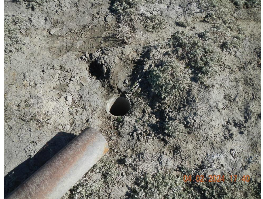
Open casing with pipe removed.
