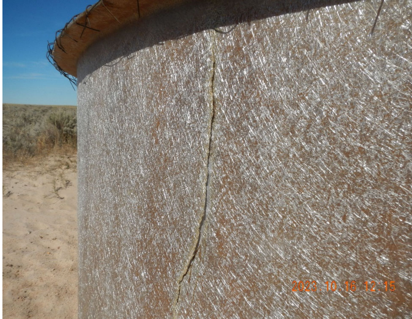
7. Split in pit wall 10/16/2023 inspection.
