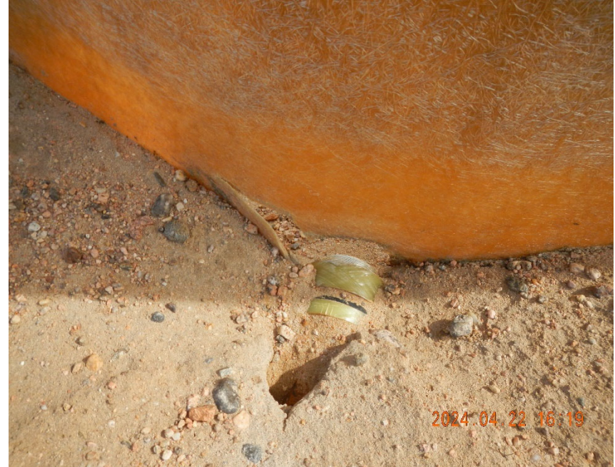
6. Hole in pit at grade level 04/22/2024 inspection.
