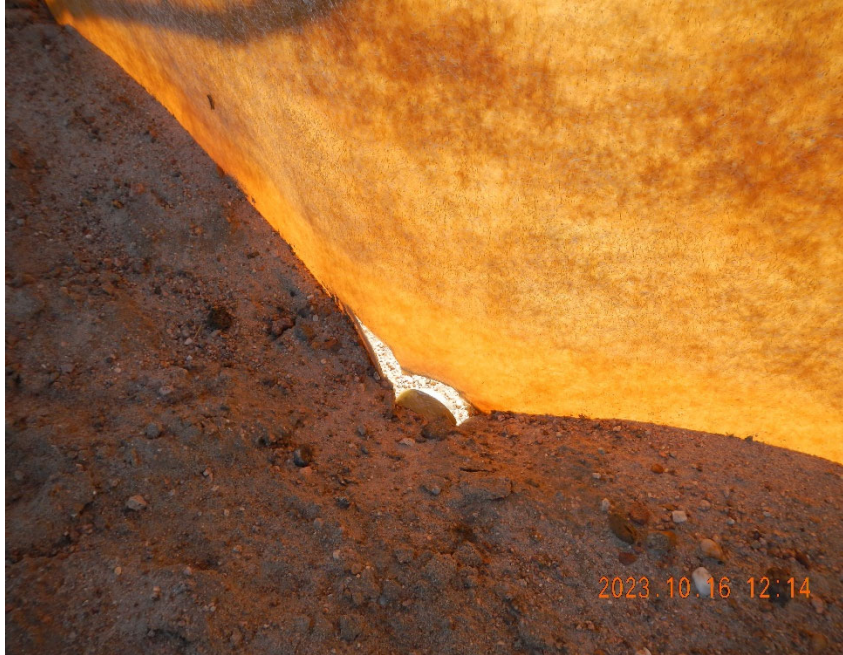
5. Hole in pit at grade level 10/16/2023 inspection.
