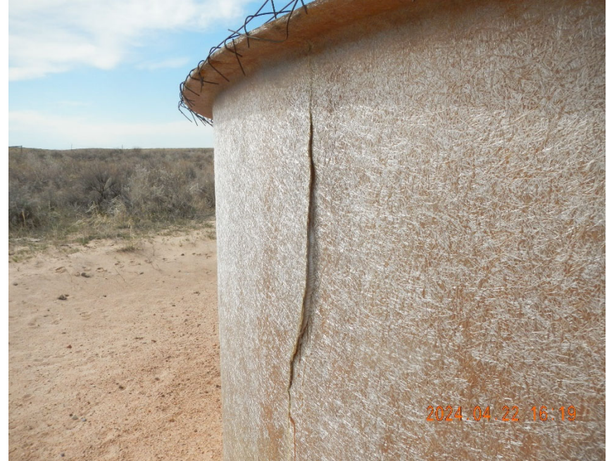
8. Split in pit wall 04/22/2023 inspection.
