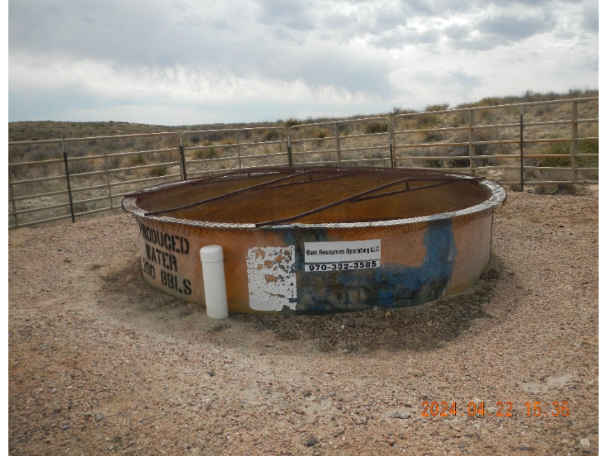
4. Produced water pit overview.
