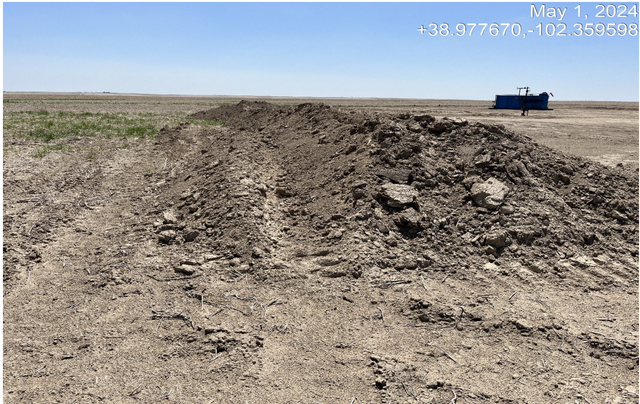
Photo 7. Northeast corner facing south. There are no stormwater controls around the location and soil pile is not stabilized.
