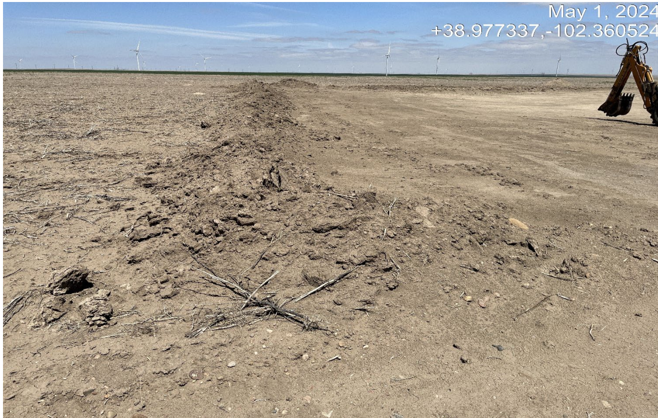
Photo 3. Facing north at the west side of the location. There is a small ~2ft. tall topsoil pile which is insufficient and not stabilized.
