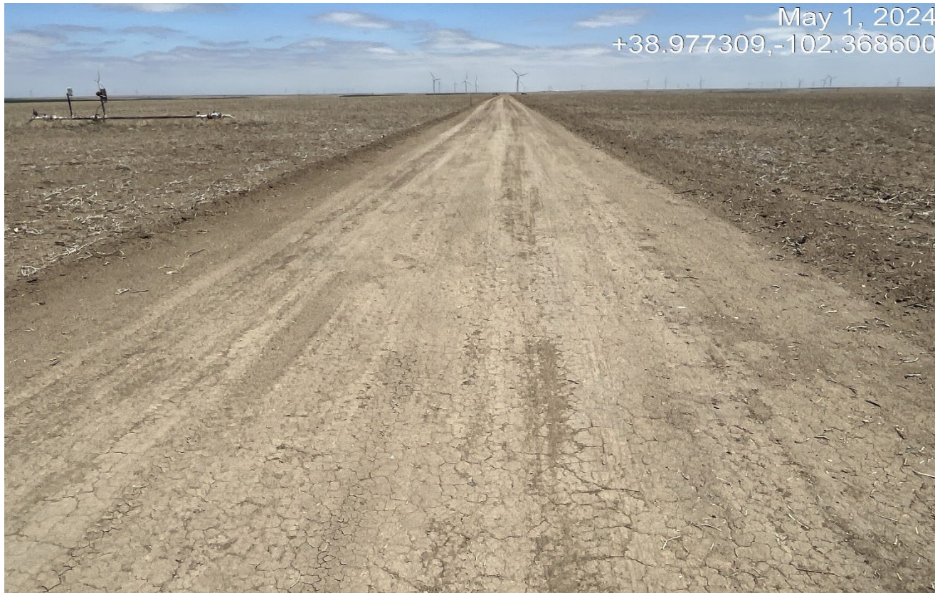
Photo 1. Facing east along the access road. Topsoil was not adequately salvaged and soils are heavily compacted along the road.
