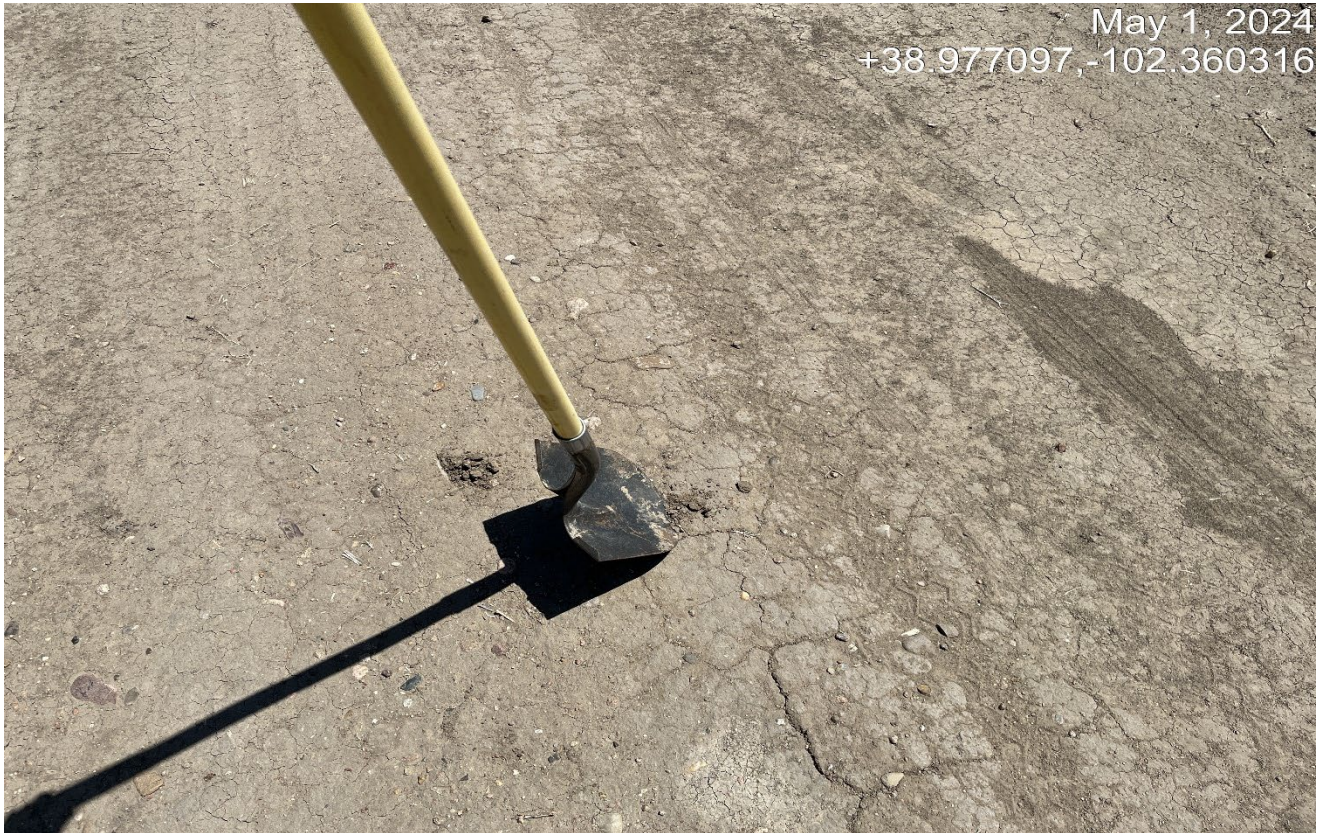
Photo 3. The soils are heavily compacted and were not protected.
