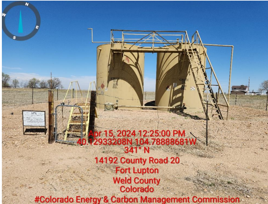
Photo 5 TNK BTRY NFPA placards faded or missing
