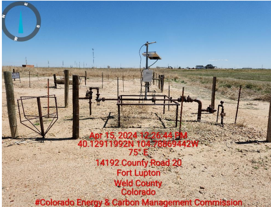
Photo 9 Meter run. Meter run not operational and has not annul calibration card. Debris: dead weeds around meter
