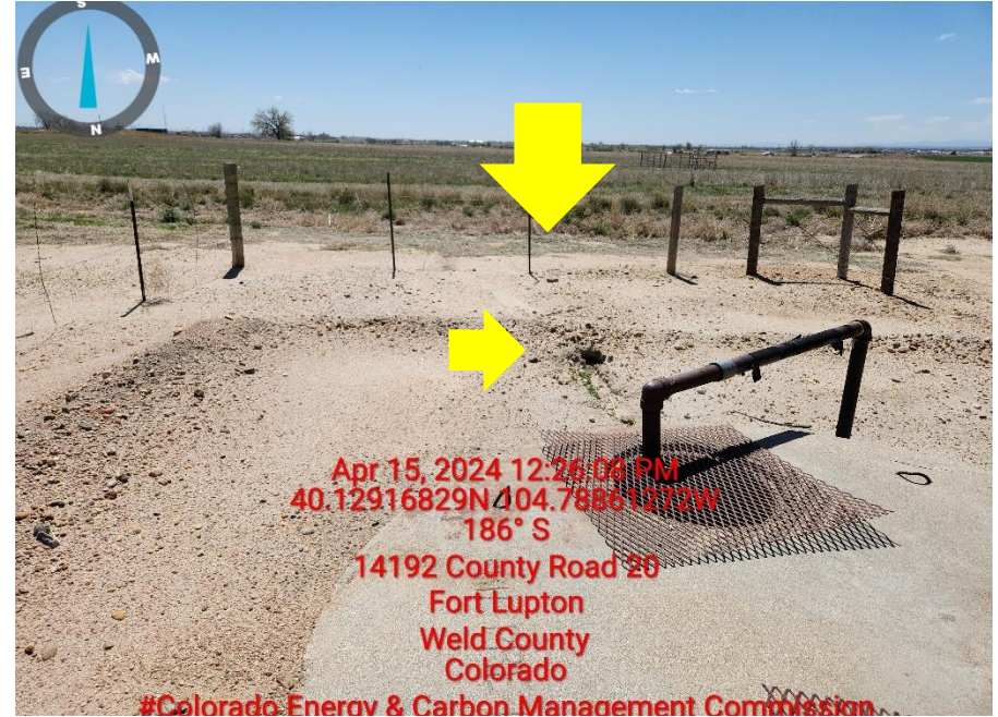
Photo 8 Hole in secondary containment allowing sediment to leave containment and run off location.
