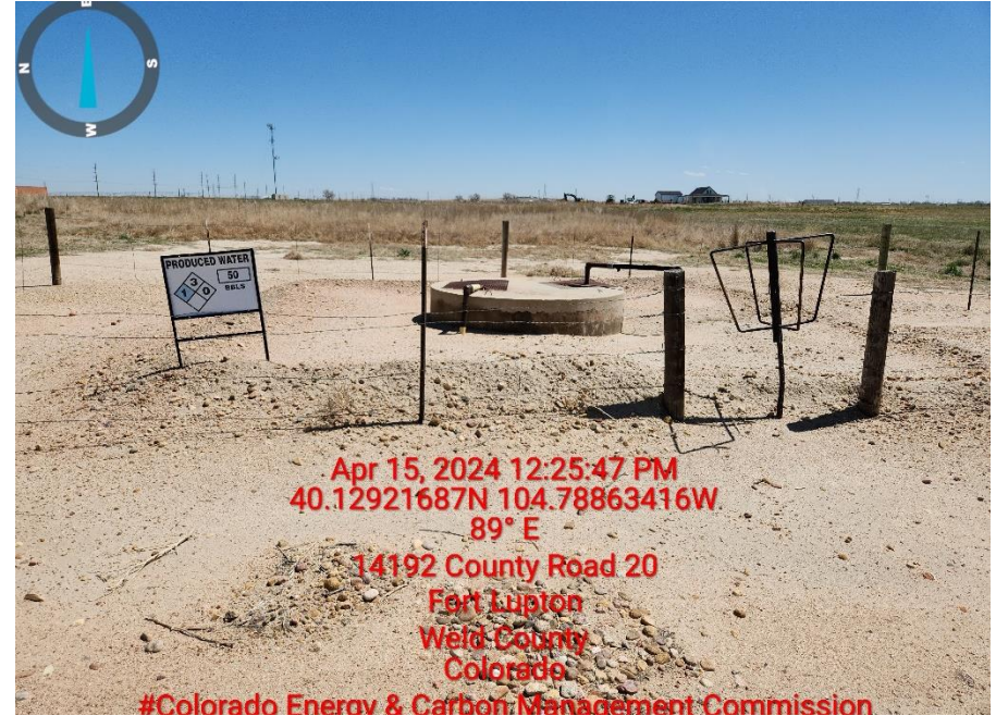
Photo 6 produced water tank NFPA placard faded
