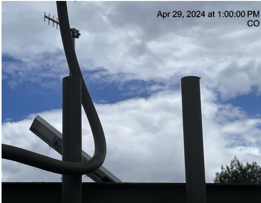
Photo # 5374 PRV & rupture disc vent lines do not comply with CECMC pressure safety device rules
