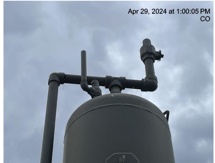
Photo # 5375 PRV vent line does not comply with CECMC pressure safety device rules
