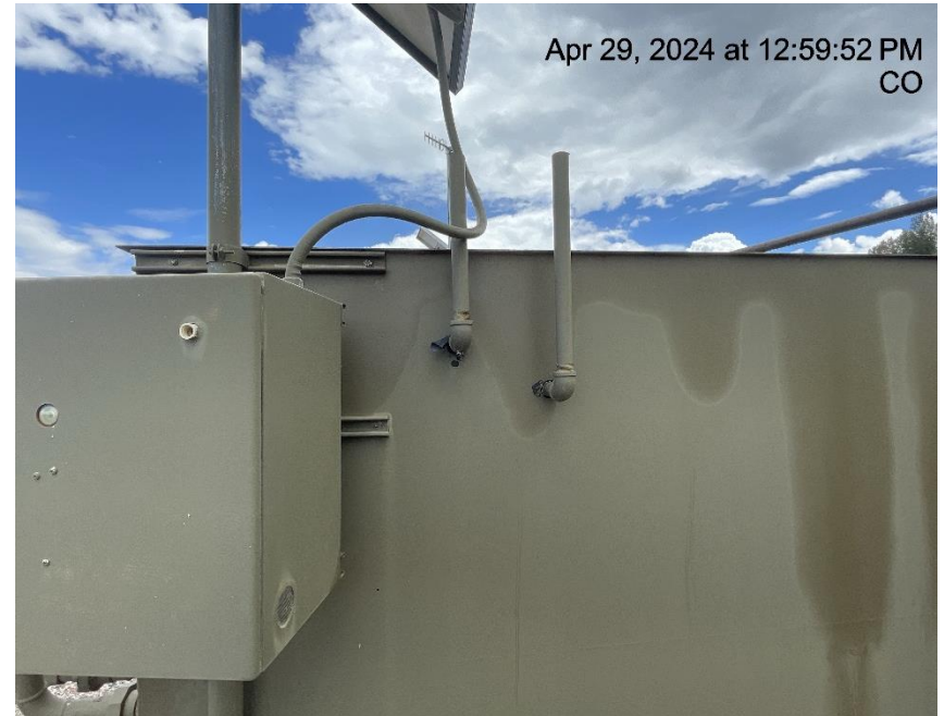
Photo # 5373 PRV & rupture disc vent lines do not comply with CECMC pressure safety device rules
