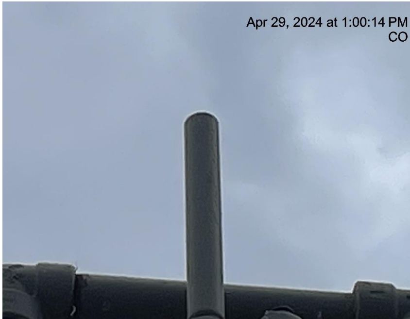
Photo # 5376 PRV vent line does not comply with CECMC pressure safety device rules
