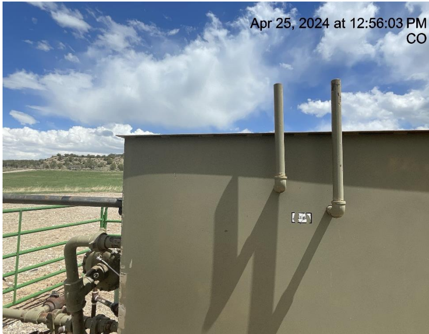
Photo # 5087 PRV & rupture disc vent lines do not comply with CECMC pressure safety device rules
