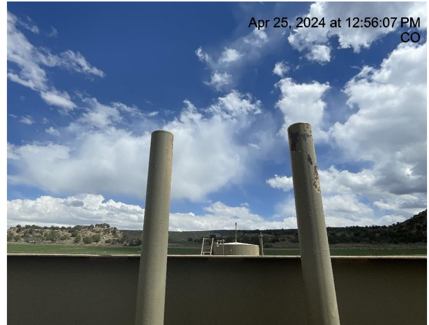
Photo # 5088 PRV & rupture disc vent lines do not comply with CECMC pressure safety device rules
