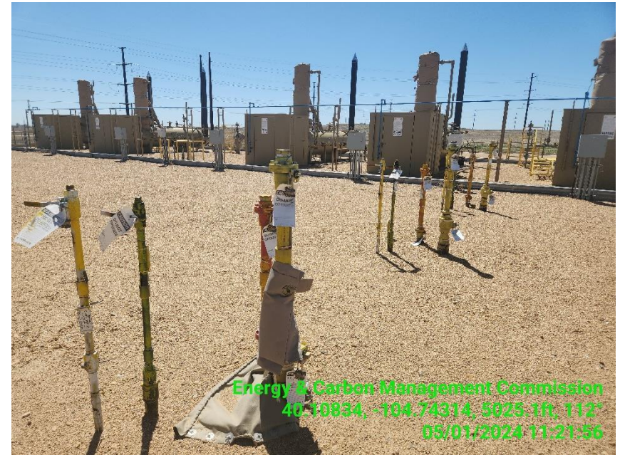
Photo 8 Horizontal Heated Separators & LOTO risers.
