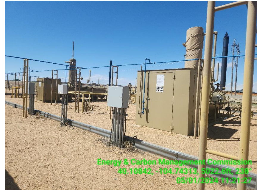
Photo 6 Horizontal Heated Separators.
