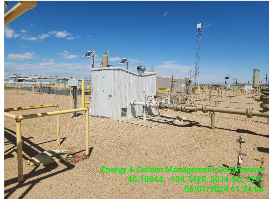
Photo 12 Gas Meter Runs, Cards indicate current calibration.
