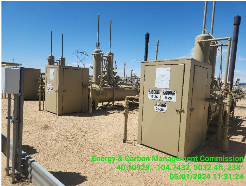
Photo 19 Horizontal Heated Separators.
