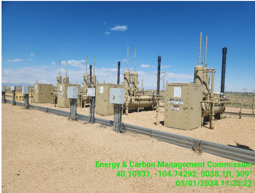
Photo 17 Horizontal Heated Separators.
