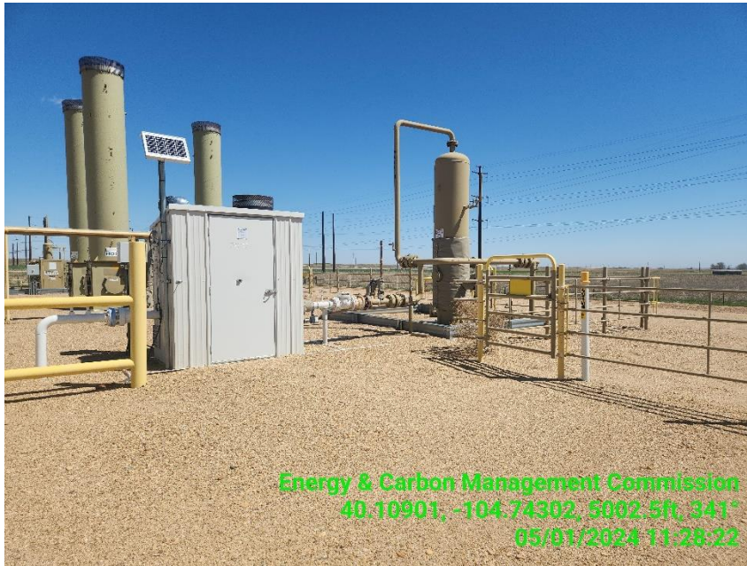
Photo 15 Gas meter run, VRT, ECDs.
