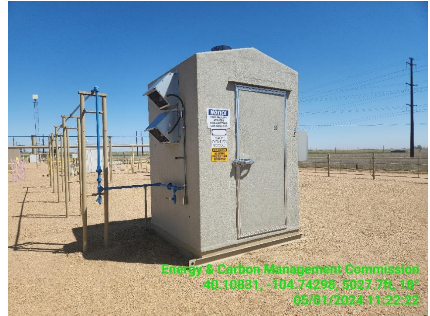
Photo 10 Compressed air dryer.
