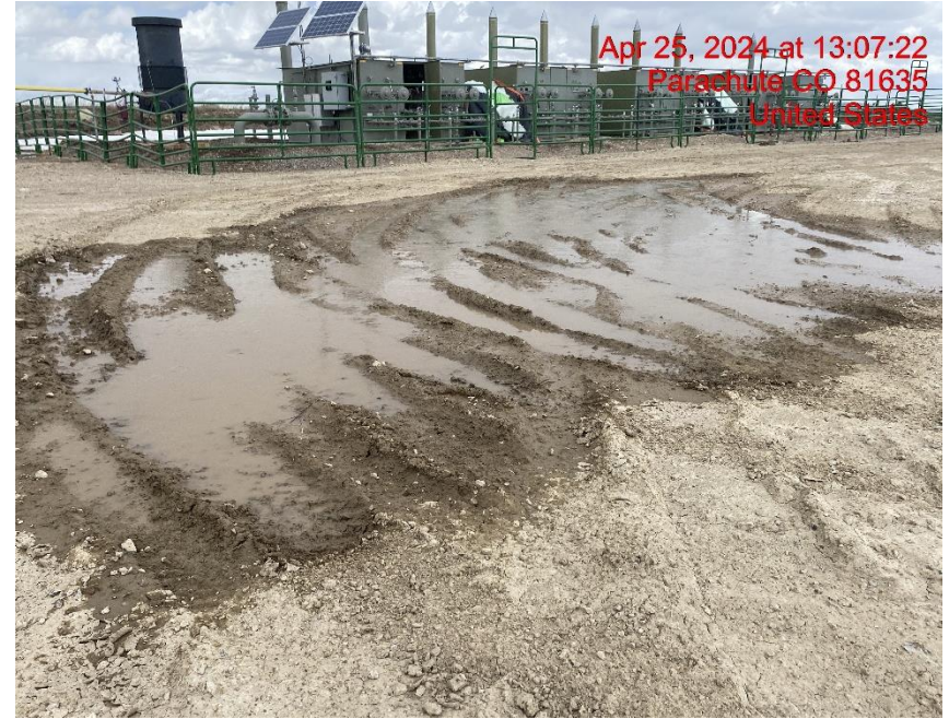
Lack of Stabilization – Photo #00891
