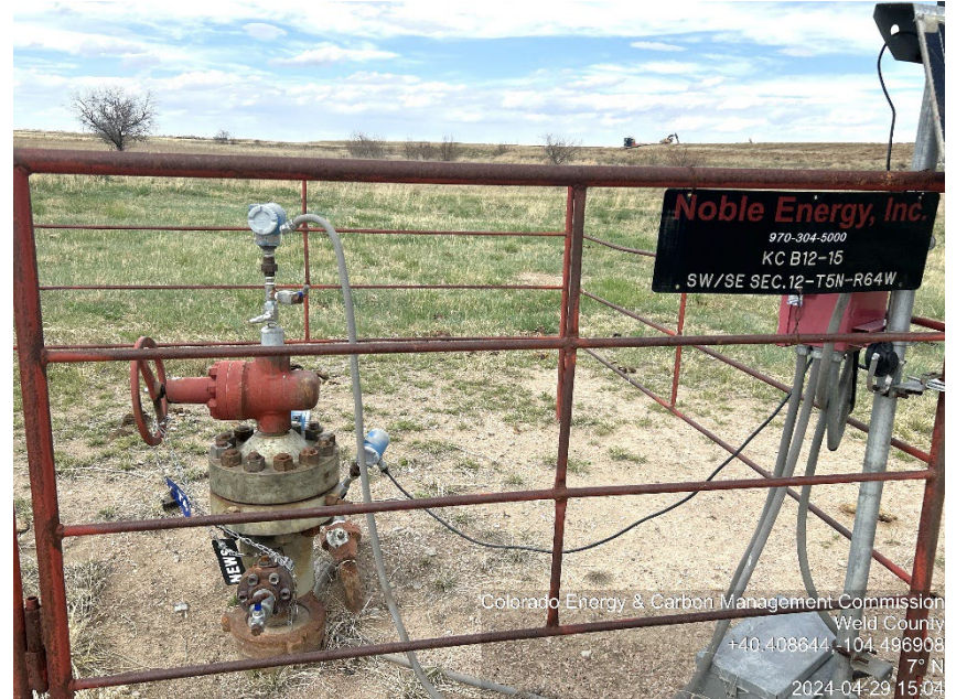
Photo #2 KC B 12-15 (123-21415) Wellsite Temporarily Abandoned | TA
