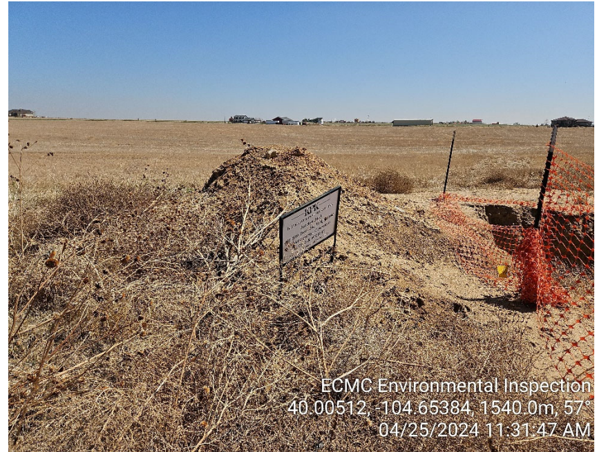
Photo 20 - Small soil stockpile. No BMPs
