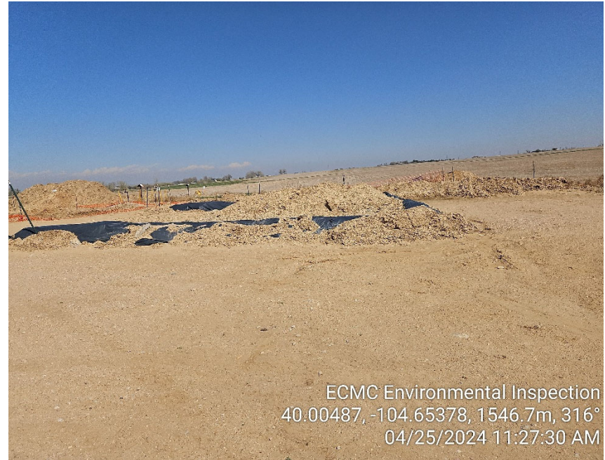
Photo 14 - Soil stockpile. Labeled contaminated. Bermed and lined; liner beginning to tear in some locations.
