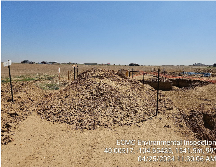
Photo 19 – Small soil stockpile. No BMPs
