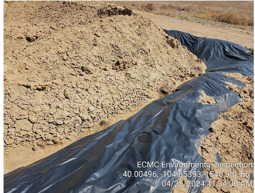
Photo 18 - Soil stockpile. Labeled contaminated. Bermed and lined; liner beginning to tear in some locations.
