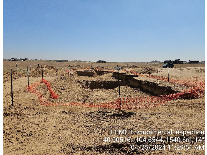
Photo 2 - Site photo; downed fencing. Soil stockpiles on either side of excavation with no BMPs.
