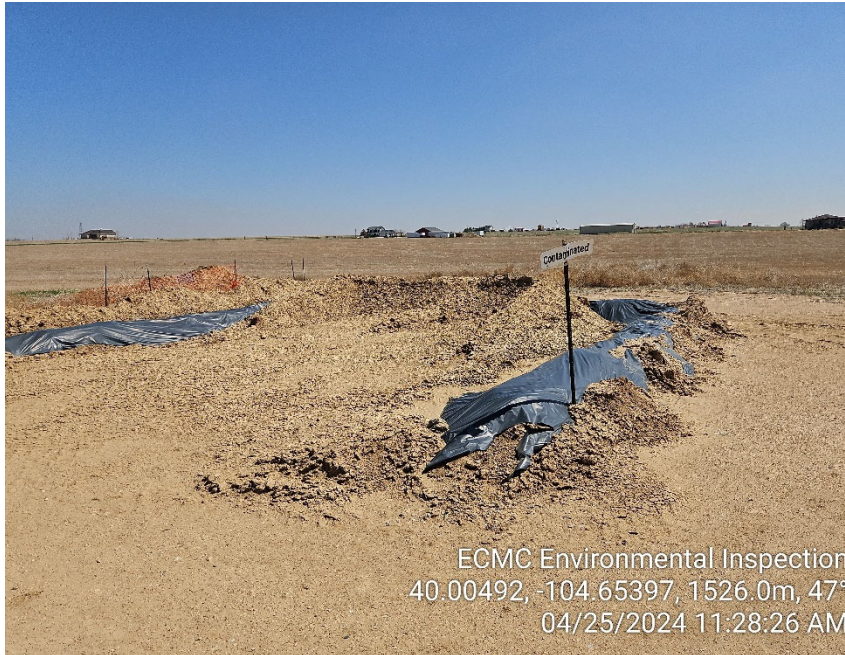
Photo 15 – Soil stockpile. Labeled contaminated. Bermed and lined; liner beginning to tear in some locations.
