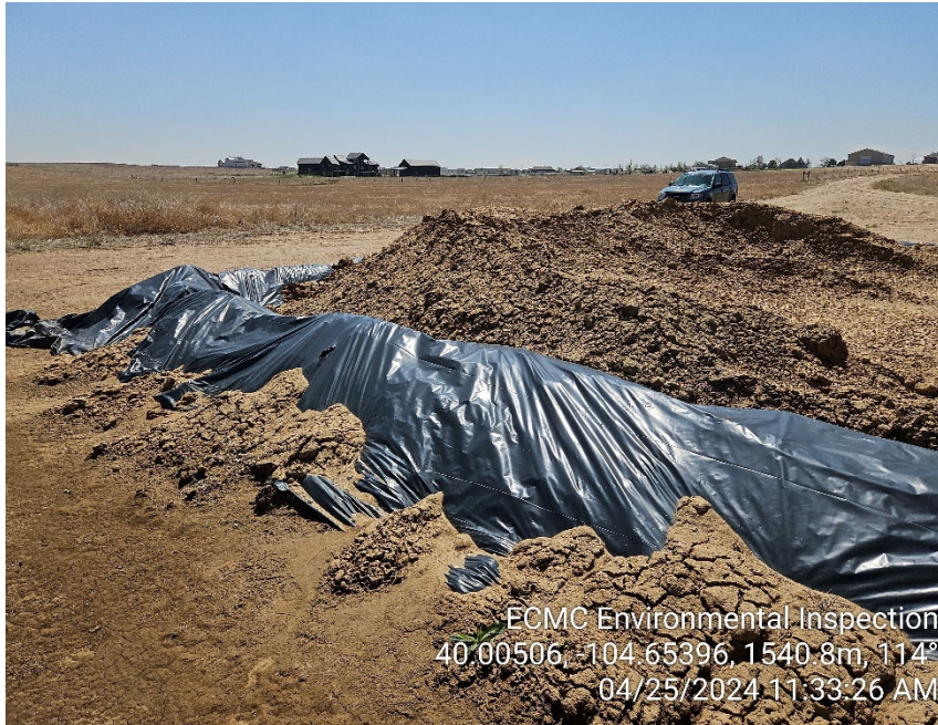
Photo 17 – Soil stockpile. Labeled contaminated. Bermed and lined; liner beginning to tear in some locations.
