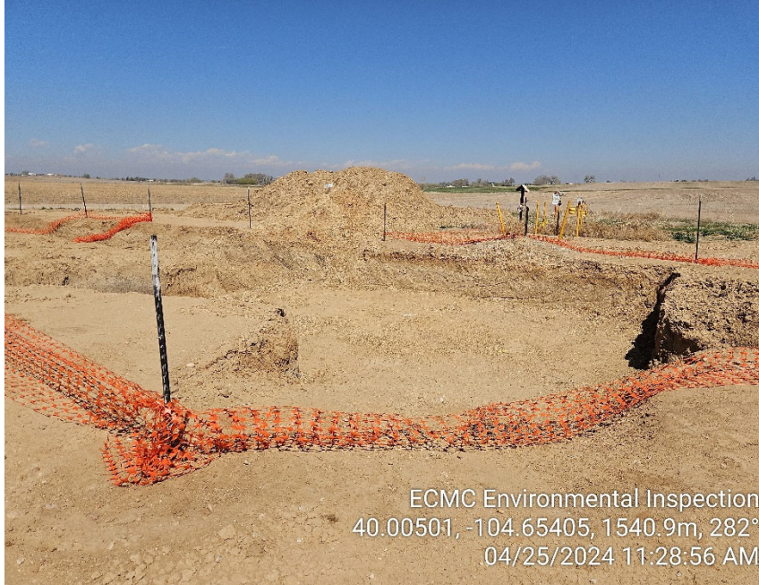
Photo 3 – Open excavation with downed fencing. Sign notes large soil stockpile in background is clean soil. Smaller soil stockpile is unmarked.
