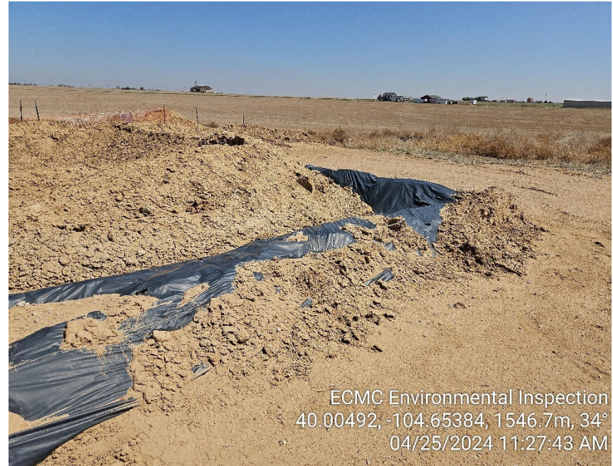
Photo 16 - Soil stockpile. Labeled contaminated. Bermed and lined; liner beginning to tear in some locations.
