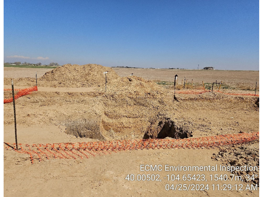
Photo 4 - Open excavation with downed fencing. Sign notes large soil stockpile in background is clean soil. Smaller soil stockpile is unmarked.
