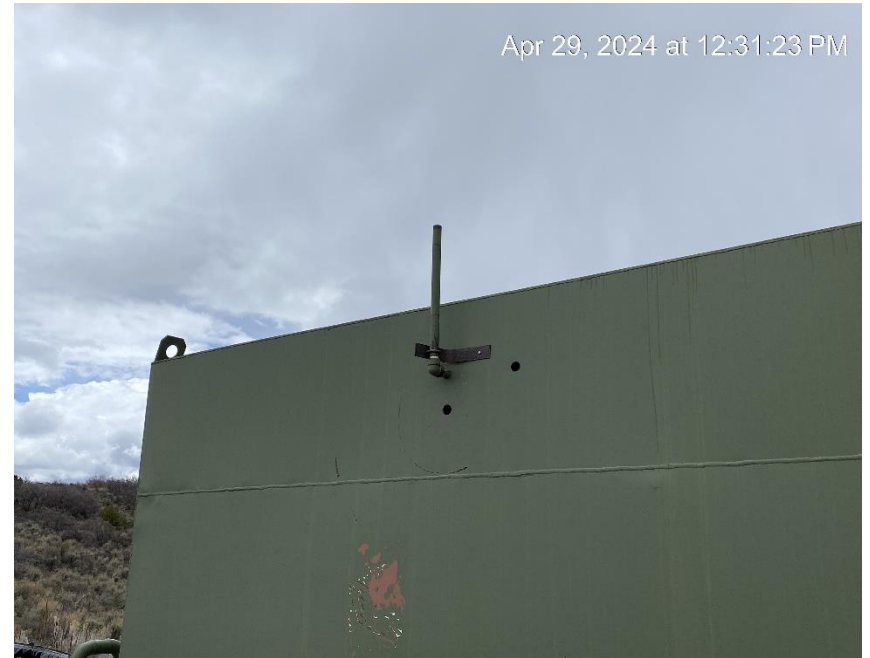
Relief riser missing rain protection
