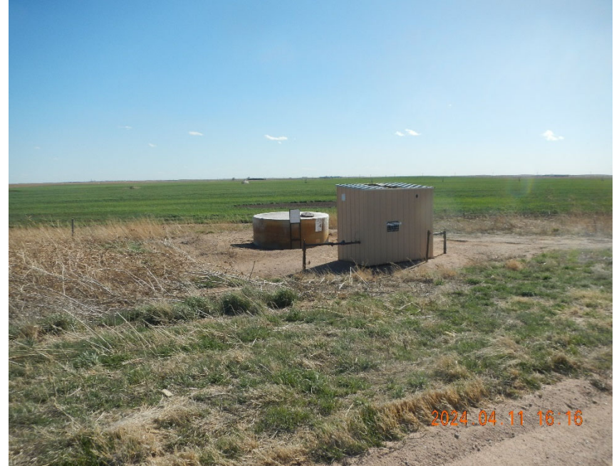
4. Remote metering location overview.
