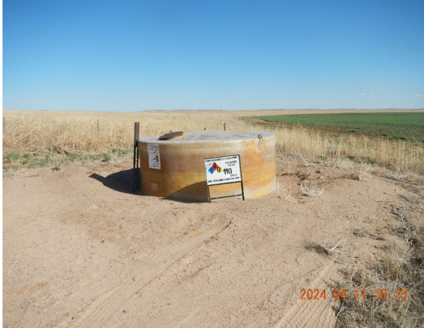
3. Produced water tank overview.
