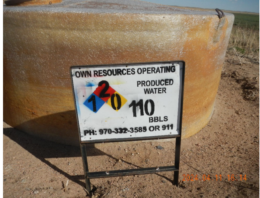
2. Content/Quantity/Hazard sign at produced water tank.
