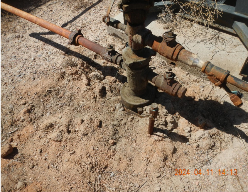
5. View of wellhead after soil turned.
