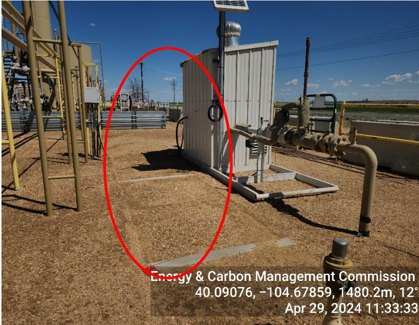
Photo 7: Unused gas meter removed
