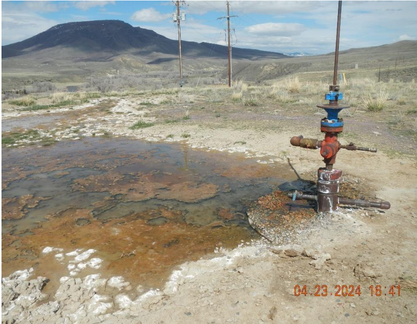
BM Federal #13-12 well head and standing water.
