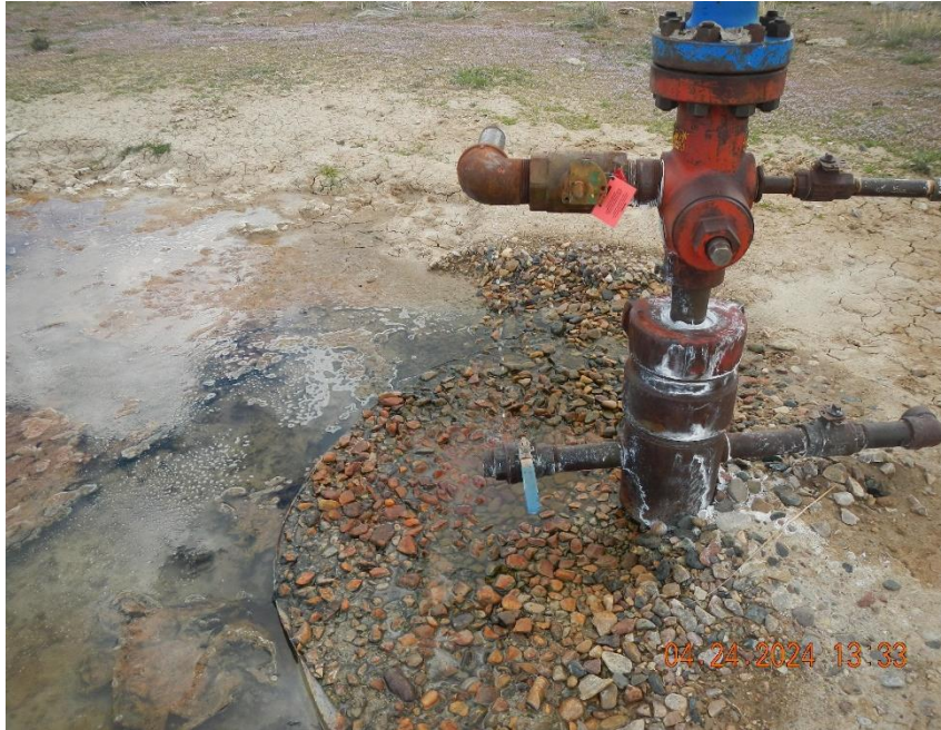
BM Federal #13-12 well head with leaking 2" valve.
