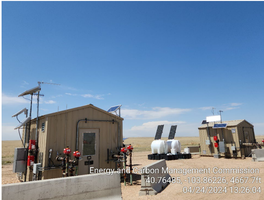
Photo 7 – Gas Lift Injection Meters
