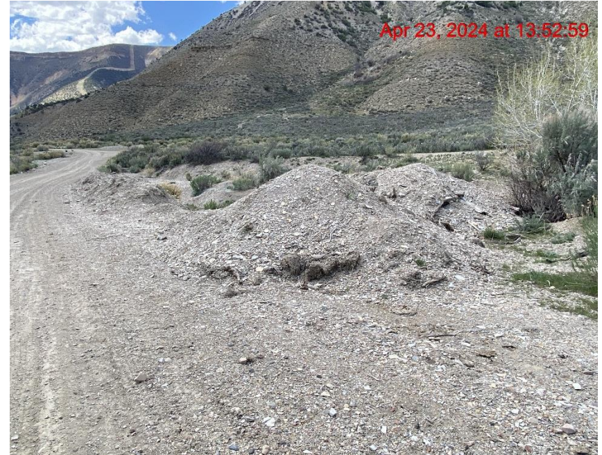
Unprotected Soil Stockpile (Access Road) – Photo #00777
