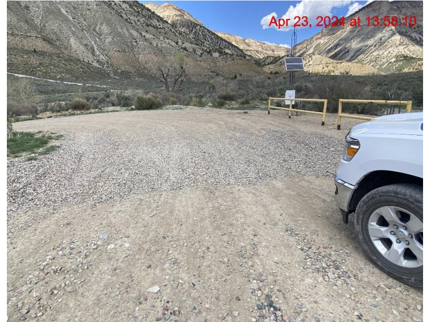
Insufficient Vehicle Tracking BMPs at Location Entrance/Exit – Photo #00786
