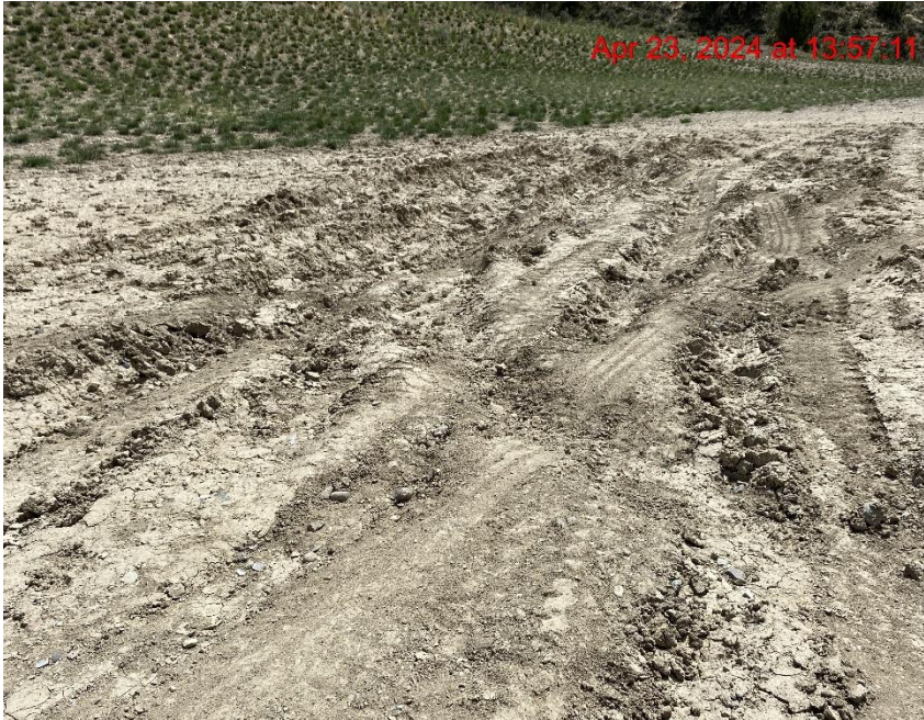
Lack of Stabilization – Photo #00784
