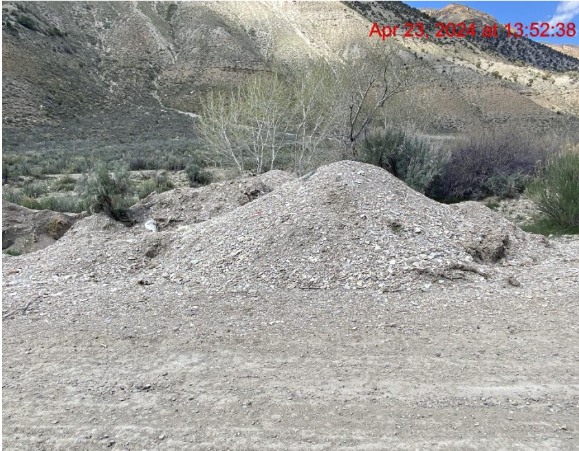
Unprotected Soil Stockpile (Access Road) – Photo #00776
