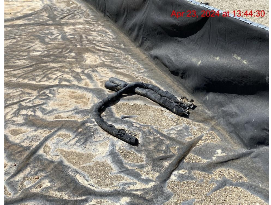
Debris in Secondary Containment – Photo #00772
