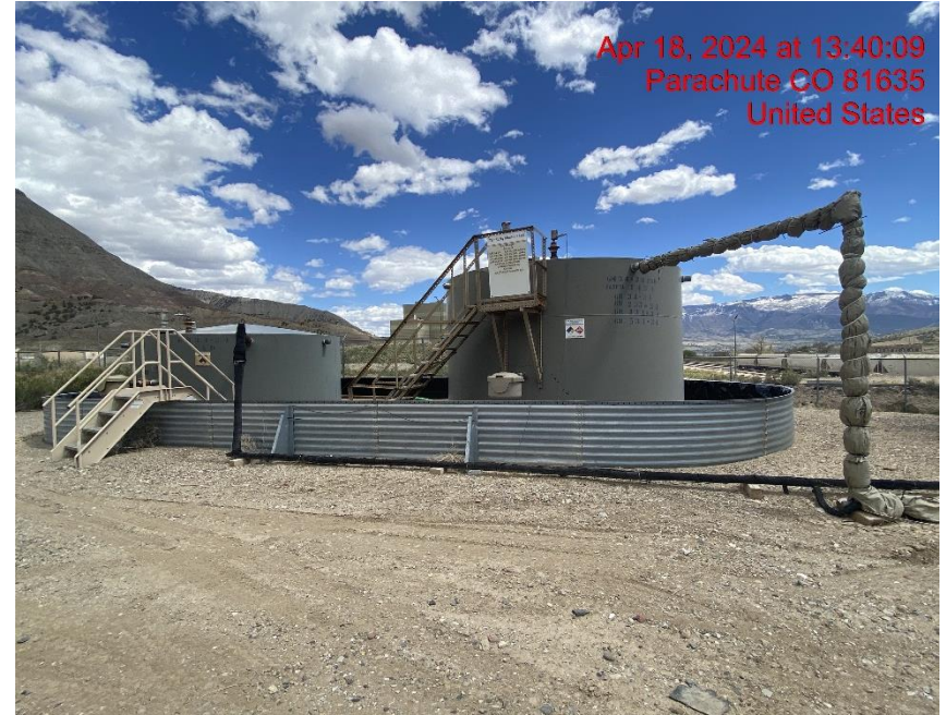
Tank Battery – Photo #00747
