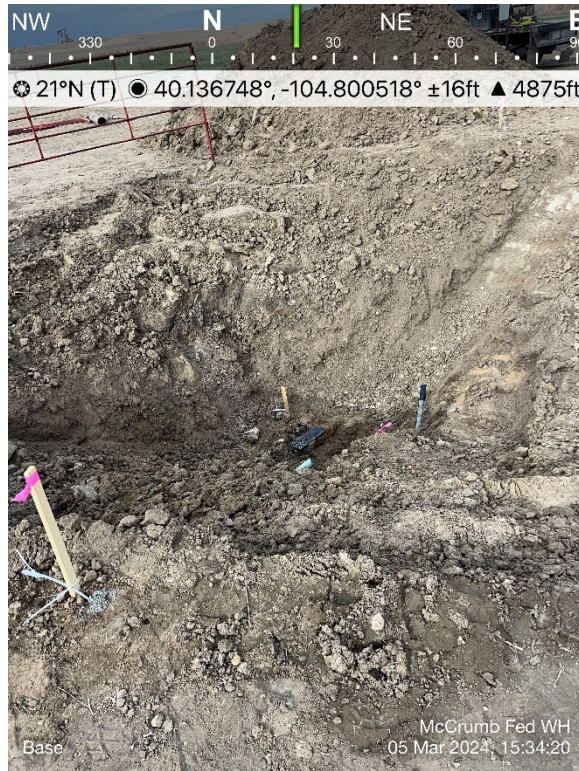
Wellhead Excavation
