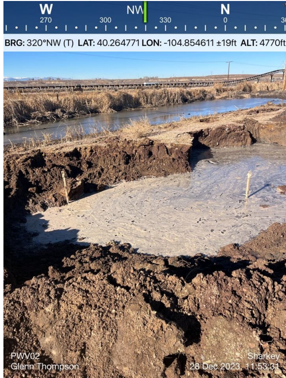
PWV 02 Excavation (Groundwater Present in Excavation)
