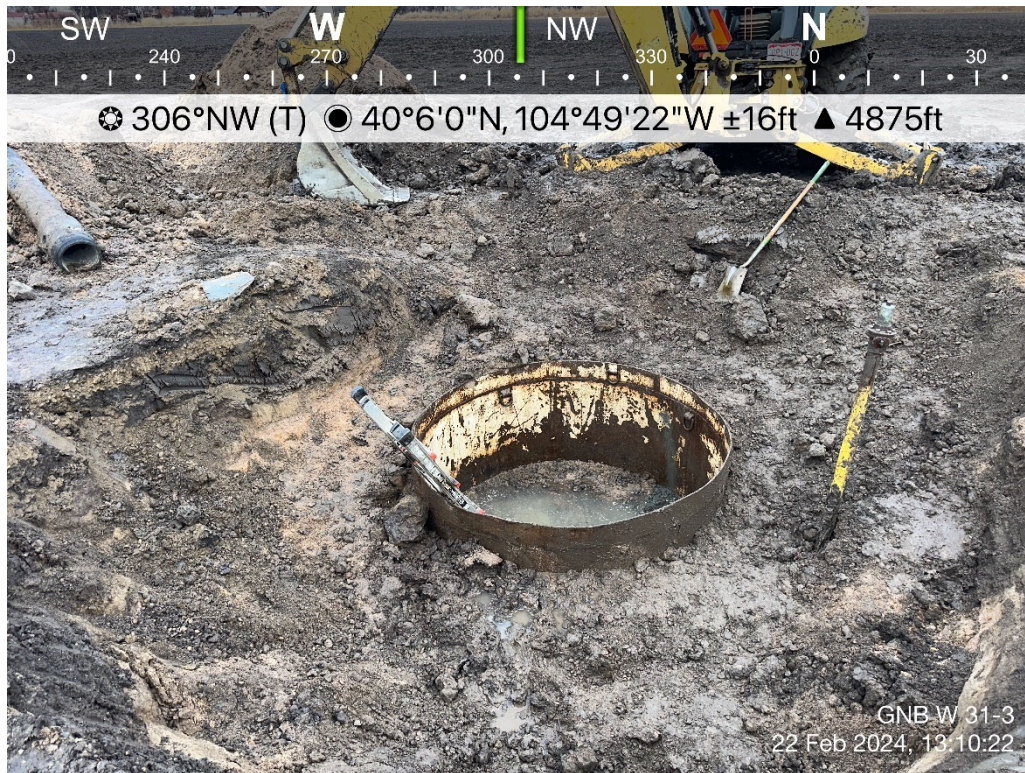
Wellhead Excavation
