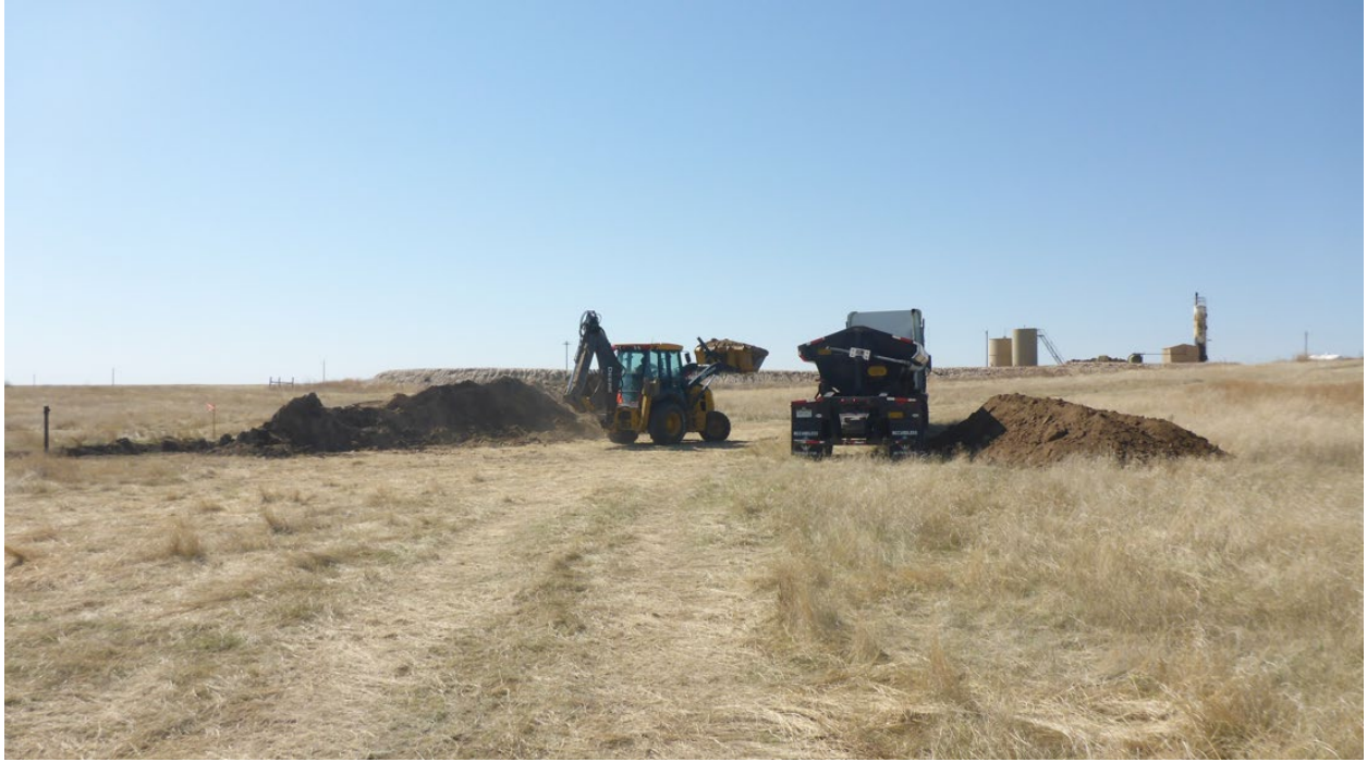
Clean topsoil staged to the west (right). Contaminated soil being loaded from the pile to the east (left).
