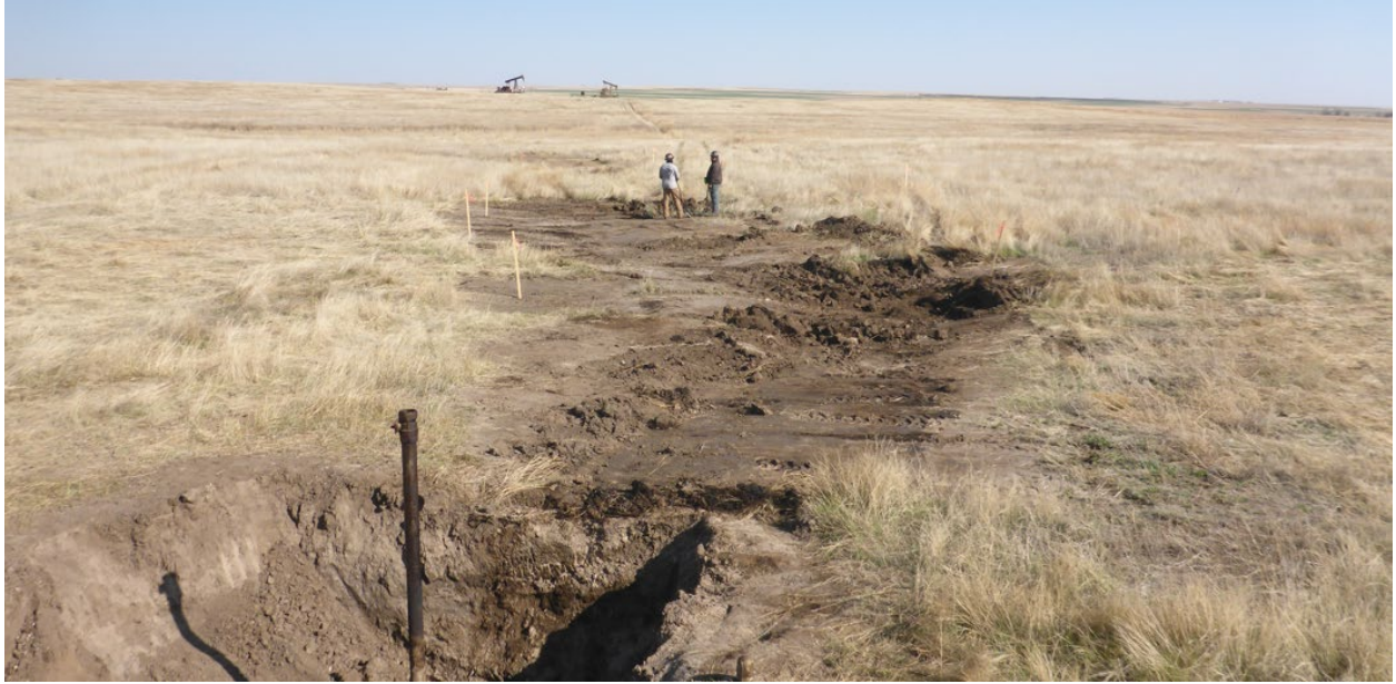
Removal of surface contamination. Lath and flag indicate area perimeter.
