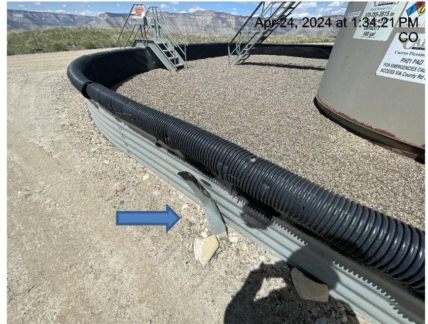
Photo # 4841 Tank containment damaged/buckling
