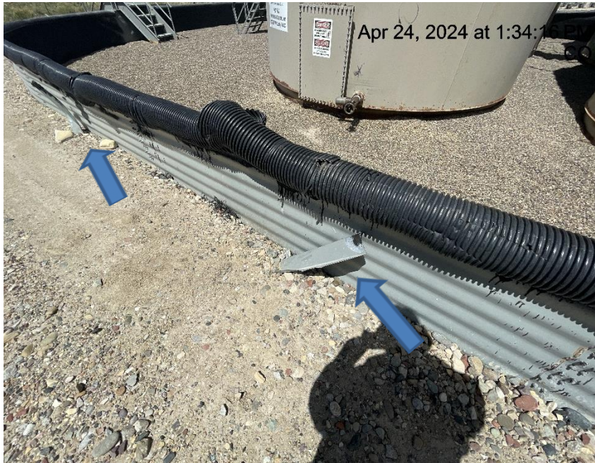
Photo # 4840 Tank containment damaged/buckling
