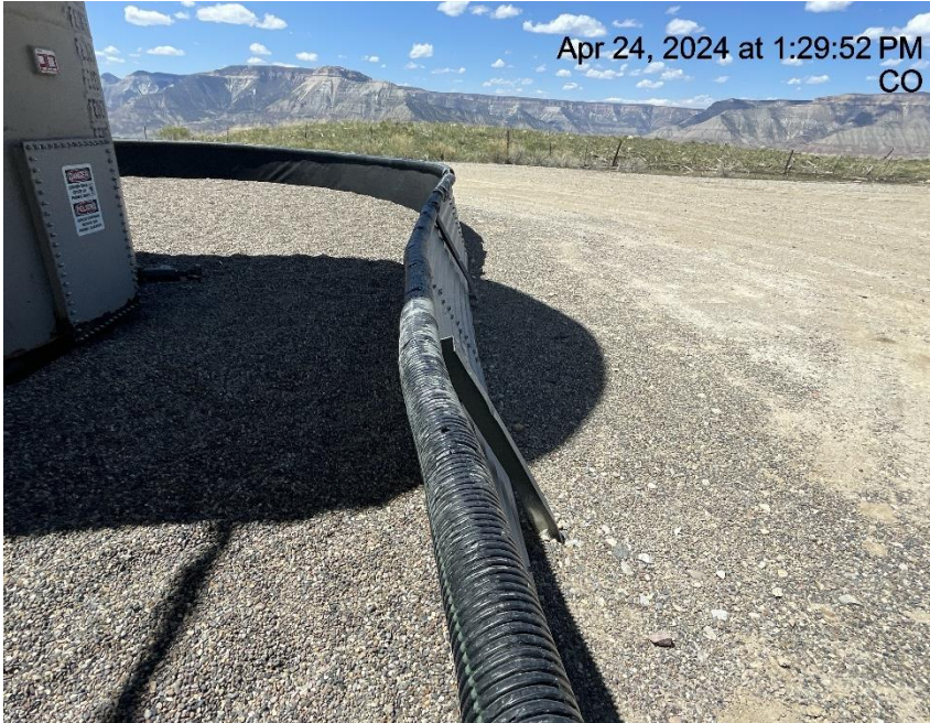
Photo # 4842 Tank containment damaged/buckling
