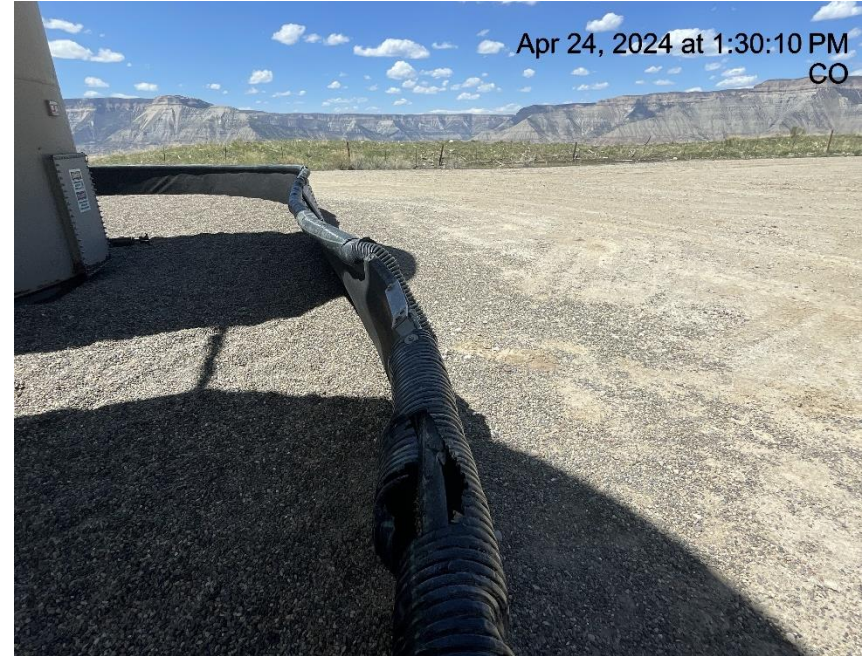
Photo # 4843 Tank containment damaged/buckling
