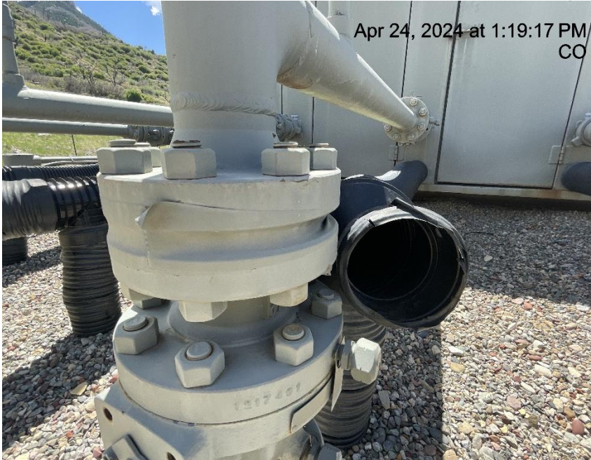
Photo # 4834 Flowline heating insulation open ended /wildlife hazard/available for entry by wildlife
