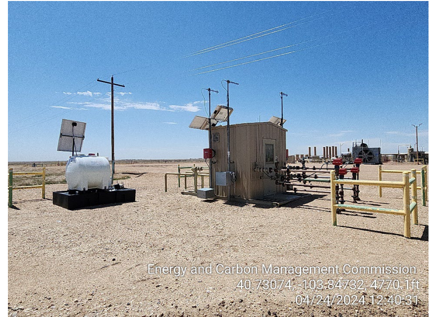
Photo 4 – Gas Lift Injection Meter House
