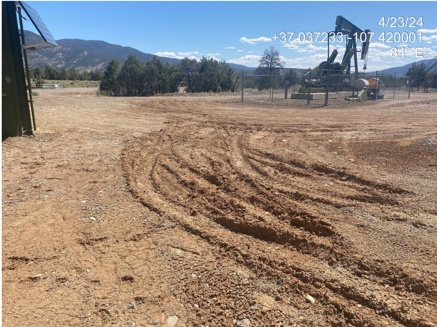
Photo 2. Rutting observed on location, additional stabilization is needed to minimize site degradation.
