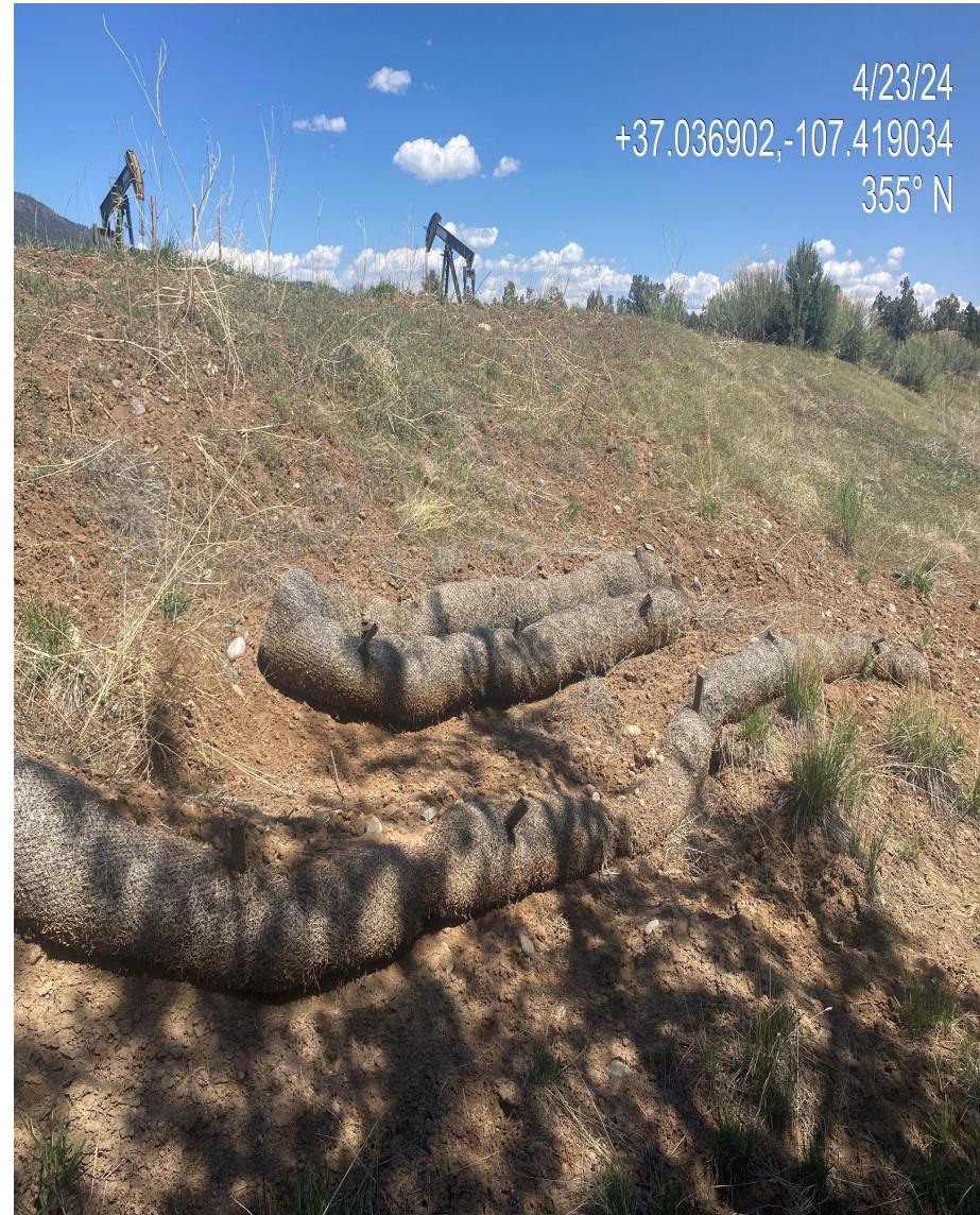
Photo 3. View of wattle BMPs that are no longer functioning and over filled with sediment.
