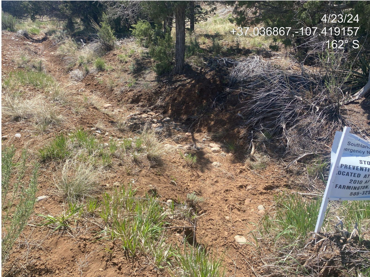
Photo 4. Inadequate/non functional storm water BMPs observed at location access point.
